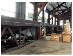
Truss Structures Between the Columns on Both Sides of the Shed
