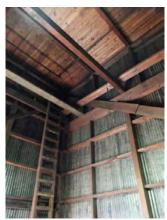
Fig.6 Diagonal Bracing
