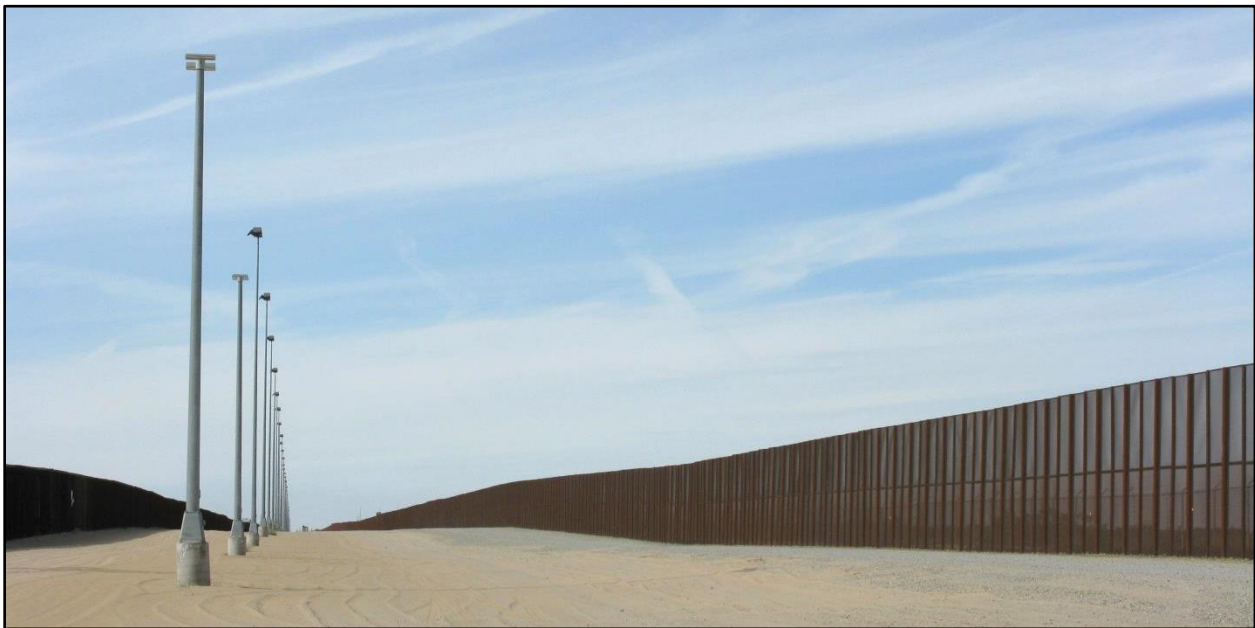
Figure 1. Trial Demonstration Site on the U.S.-Mexico Border: Daytime. Photo taken from the east end of the 7.2 mile area between poles 205 (not pictured) and 204 (pictured, front), looking west. The QMH luminaires are mounted on the poles at a height of 64 ft and the LED luminaires are mounted at 40 ft—a difference that is visible in this image. The primary fence is on the left and the secondary fence is on the right.
