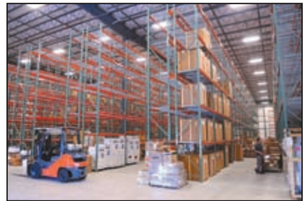
F.W. Webb Co.'s newly constructed 'green' facility in Waterford, Conn., was built with energy efficient systems to be more environmentally friendly and could save up to $60,000 annually on energy bills.
