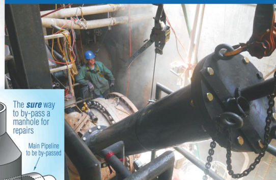
Plugging a pressurized pipeline
