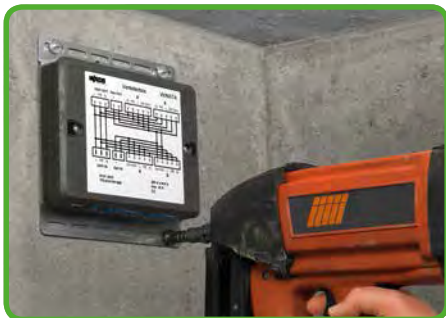
Securing the mounting plate with WINSTA® Distribution Box to the wall (e.g., via stud gun).
