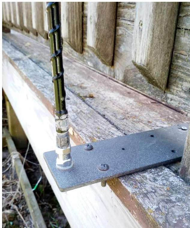
Mounting bracket for Hamstick™ Antenna
