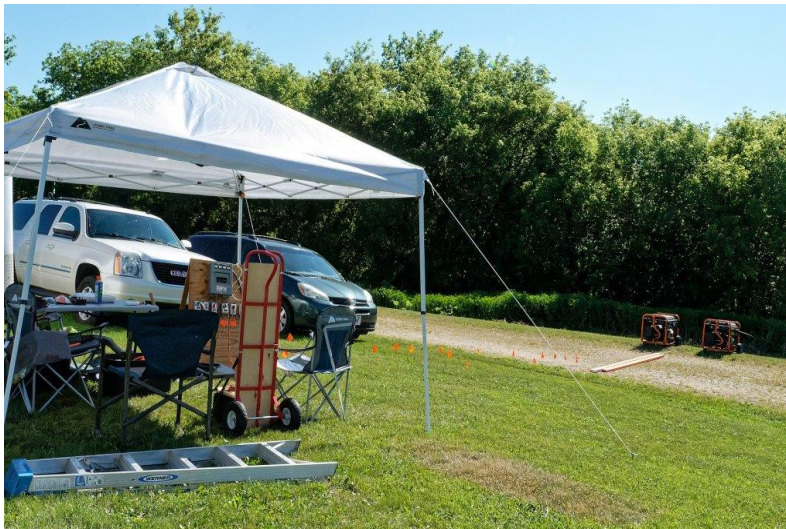
Emergency power supplied by a pair of generators, and our custom power distribution panel
