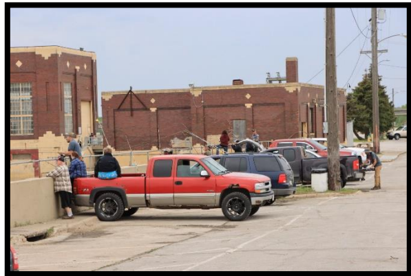
Figure 4-6. Levee Wall in Market Street Parking Lot
