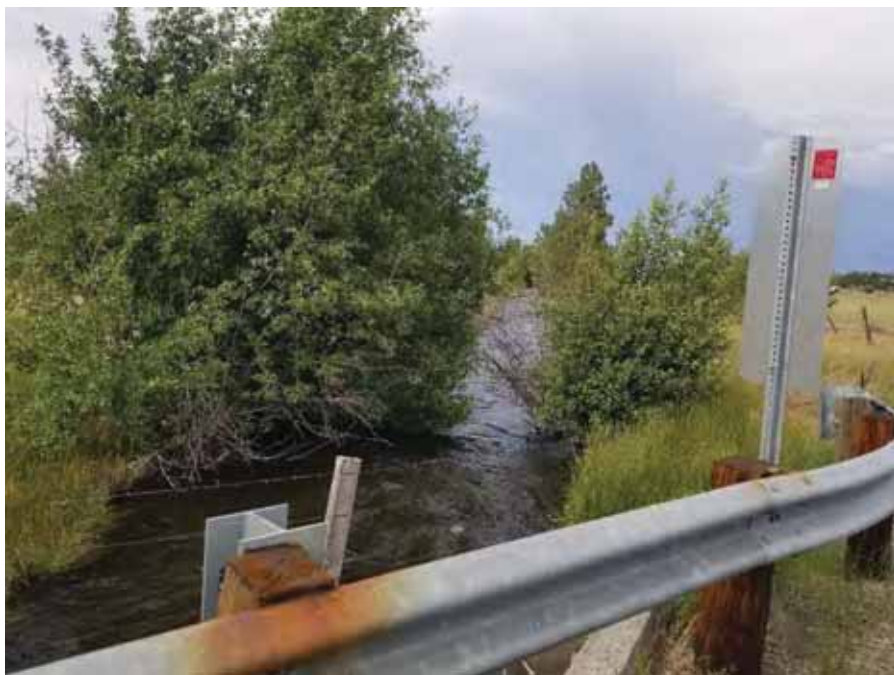
Figure 4-18. View of West Branch Lateral Crossing Pinehurst Road Looking Northeast in 2017.
