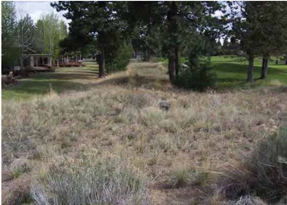
Figure 6-3. A Section of the Bend Feed Canal after a Piping Project.
