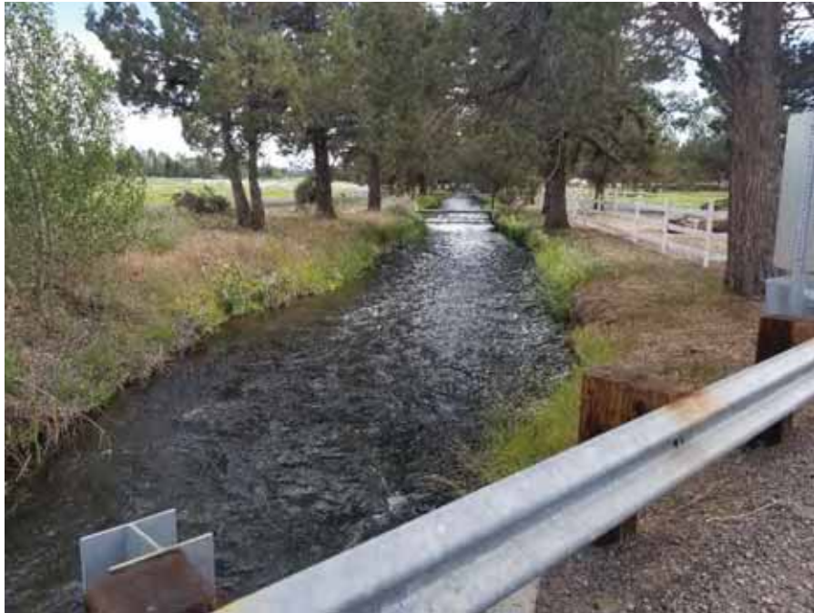
Figure 4-17. View of West Branch Lateral Looking Southwest where it Crosses Pinehurst Road in 2017.
