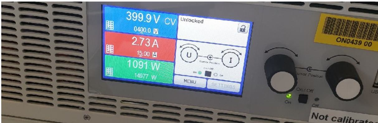
Figure 23. DC Power Supply Reading @ 1 kW.
