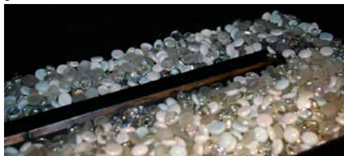
Figure 30. Completed glass bead installation. (Note: place glass beads on top of mesh pilot cover.
