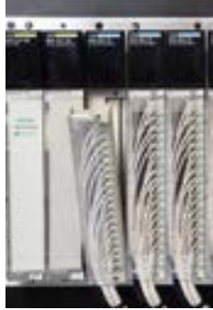
Remove existing Field Wiring adapters
