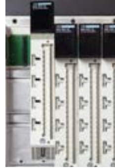
Remove existing controller cards
