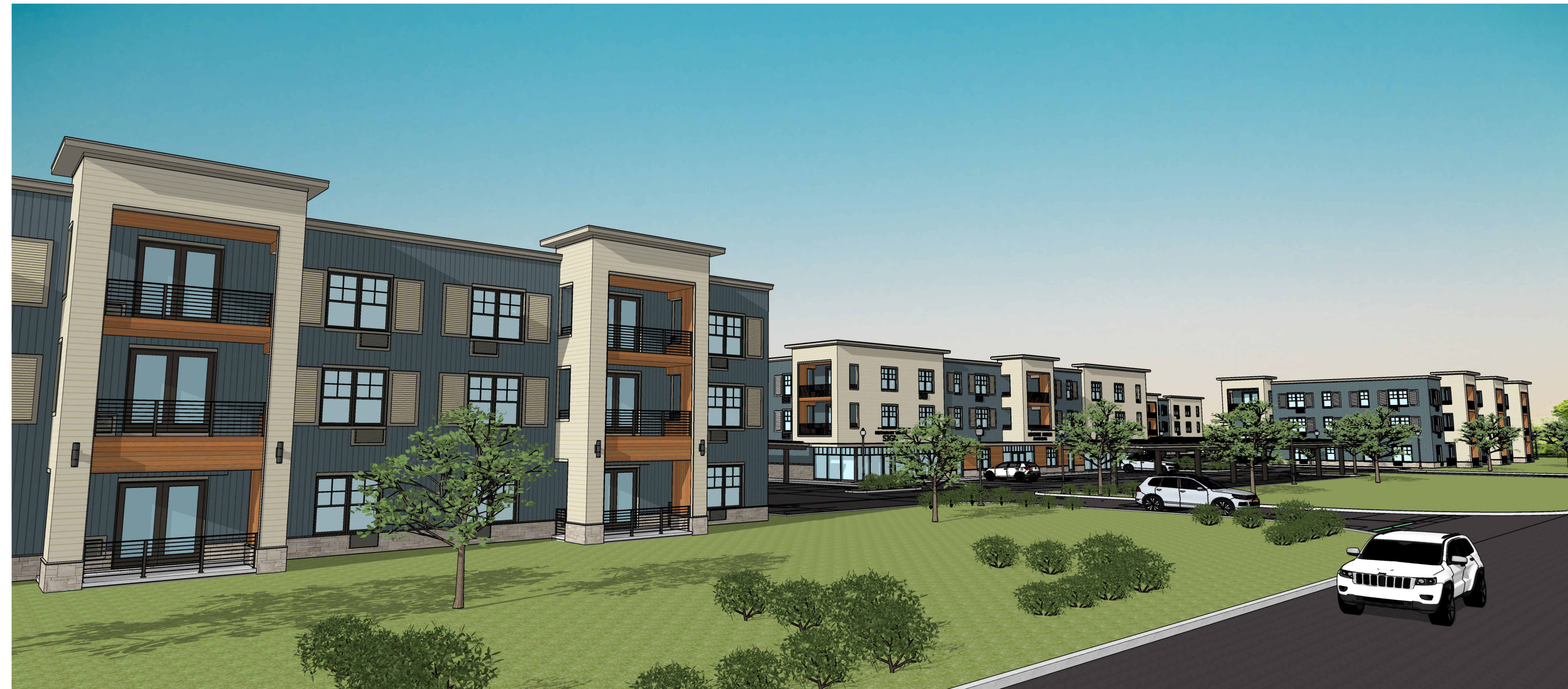
VIEW FROM OLD LIVERPOOL ROAD
