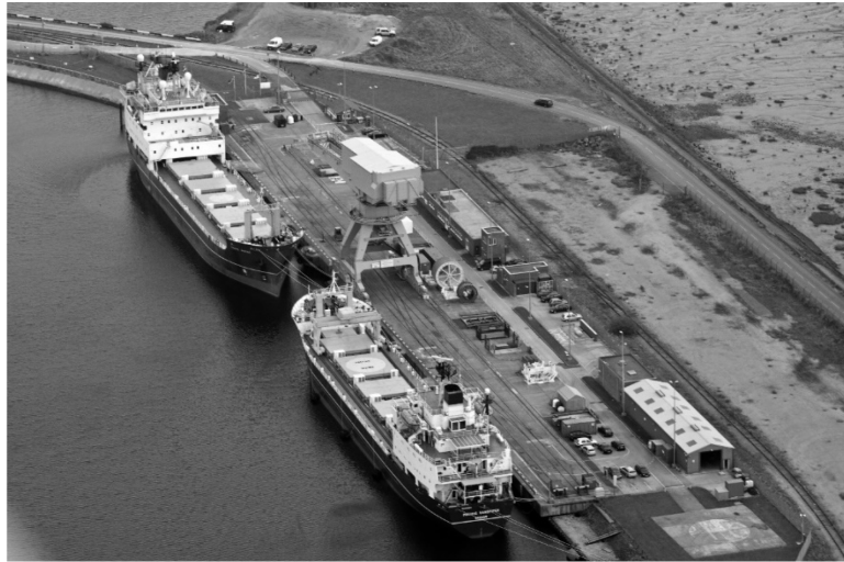
Figure 2. Aerial view of Barrow Marine Terminal
