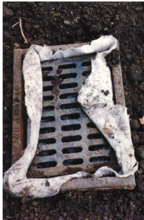
Figure 6: Catchbasin with geotextile to protect storm sewer pipes from sediment contamination
