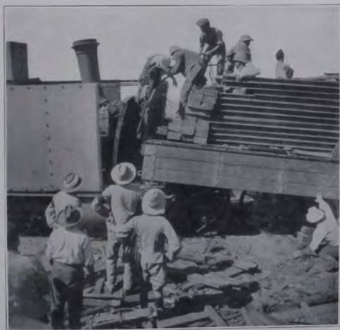
FIG. 2.—Accident illustrating strength of rail and sleeper type of armouring.
