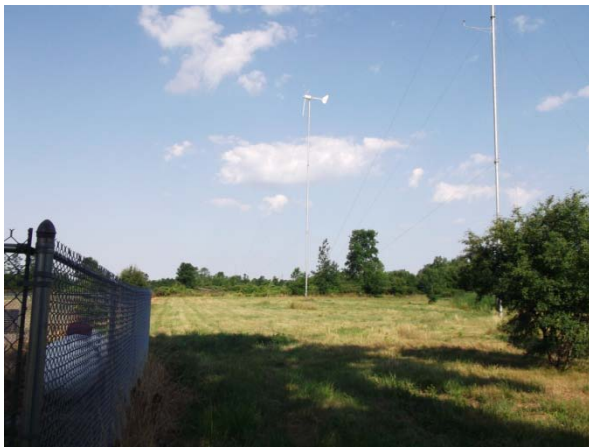
Figure 3-16. Small Wind Project (two turbines), Renewable Energy Program Area
