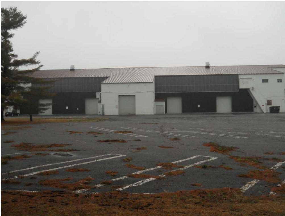
Figure 3-7. Solar Wall Collectors (exterior view) at Monitored Project, Renewable Energy Program Area
