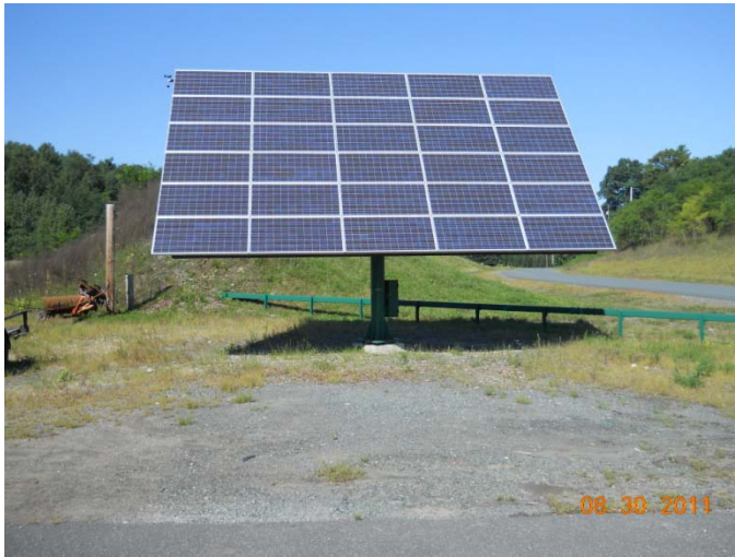
Figure 3-8. Tracking PV Array, Renewable Energy Program Area
