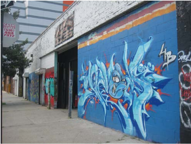
1. View of the east side of the site building along Gerard Avenue.
