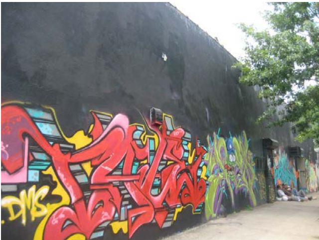
3. View of the north side of the subject property building along East 146th Street.
