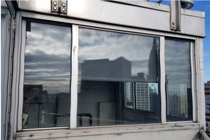
PENTHOUSE RIBBON WINDOWS UPPER LEVEL, NORTH SIDE LOOKING WEST
