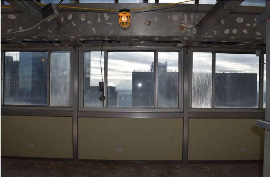
PENTHOUSE RIBBON WINDOWS LOWER LEVEL, LOOKING EAST
