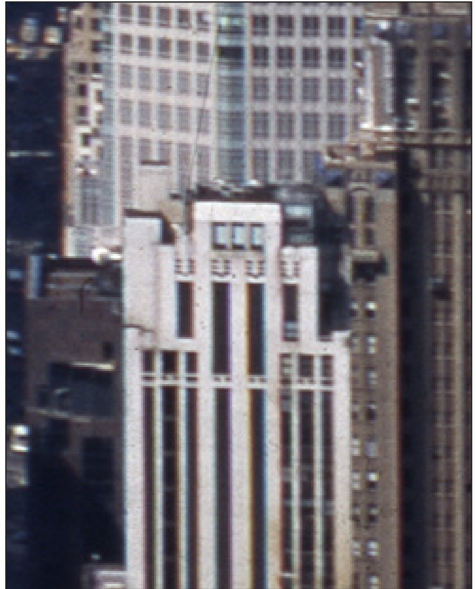
1980 DETAIL - LOOKING NORTH AT SOUTH ELEVATION
