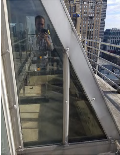
SKYLIGHT UPPER LEVEL, LOOKING NORTH
