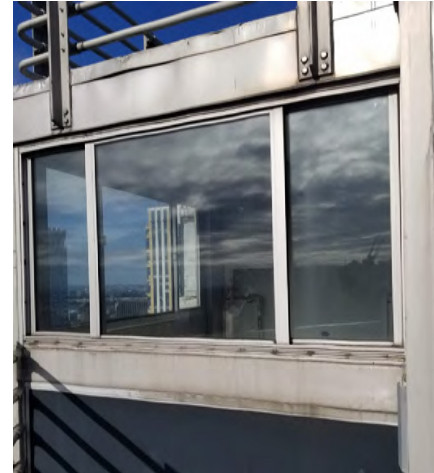
PENTHOUSE RIBBON WINDOWS UPPER LEVEL, NORTH SIDE
