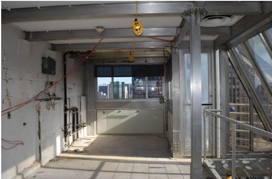
PENTHOUSE RIBBON WINDOWS UPPER LEVEL, LOOKING NORTH
