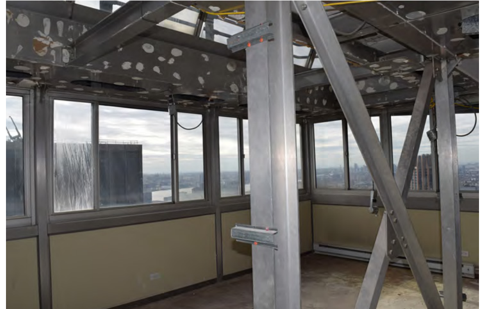
PENTHOUSE RIBBON WINDOWS LOWER LEVEL, LOOKING SOUTHEAST
