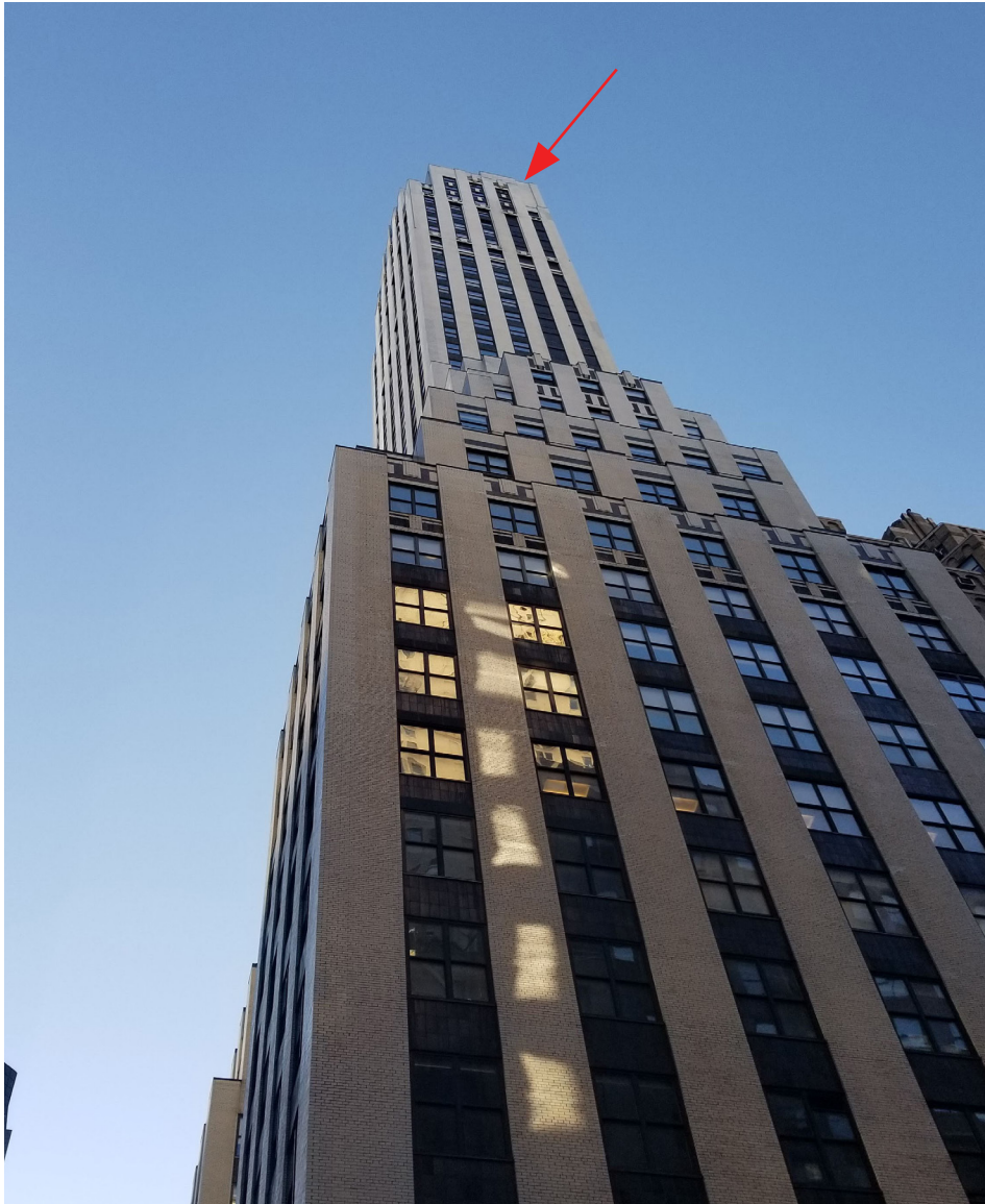
275 MADISON AVENUE LOOKING UP FROM MADISON AVENUE & EAST 40th STREET
