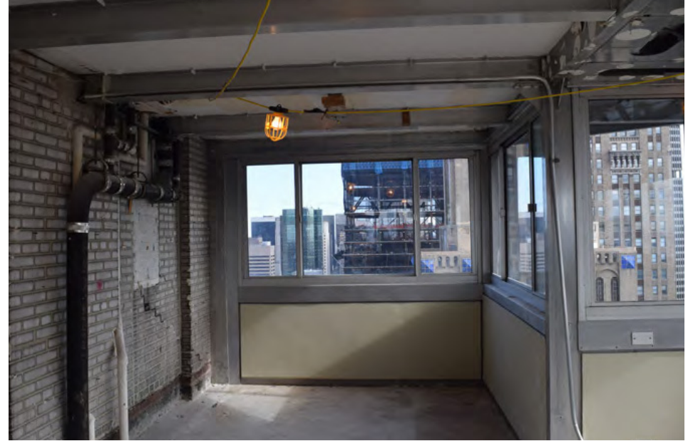
PENTHOUSE RIBBON WINDOWS LOWER LEVEL, LOOKING NORTH
