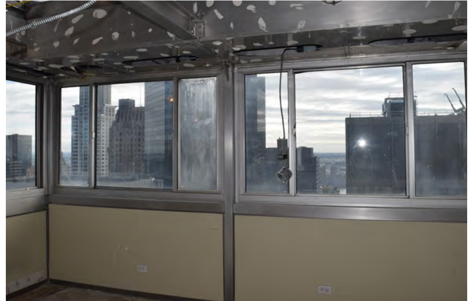
PENTHOUSE RIBBON WINDOWS LOWER LEVEL, LOOKING EAST
