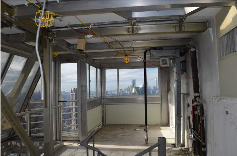
PENTHOUSE RIBBON WINDOWS UPPER LEVEL, LOOKING SOUTH
