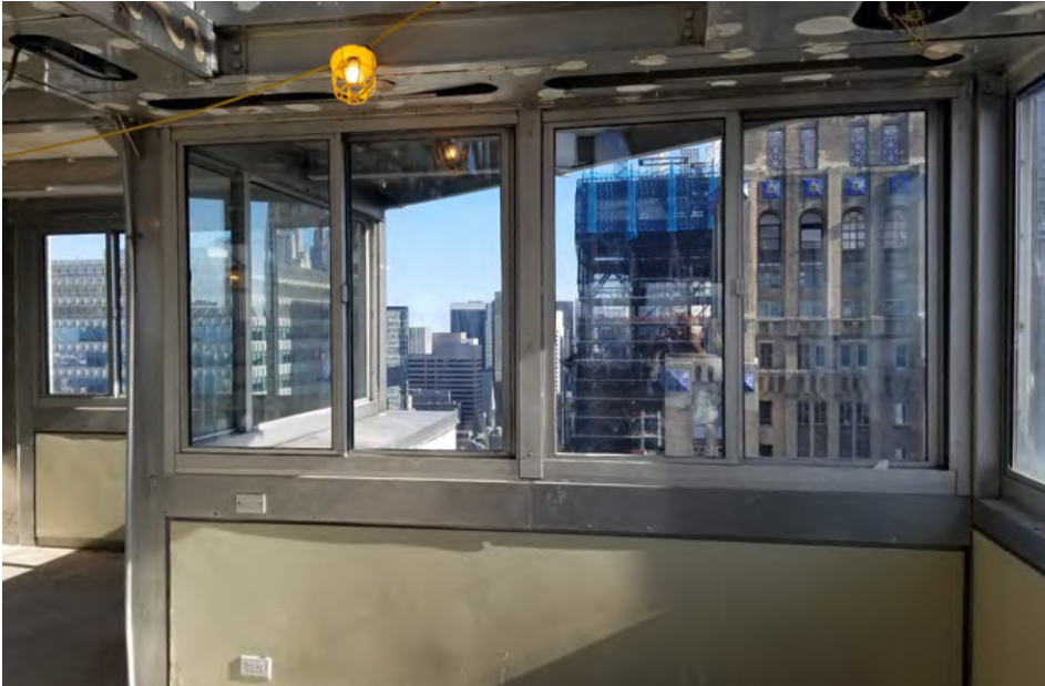
PENTHOUSE RIBBON WINDOWS LOWER LEVEL, LOOKING NORTH
