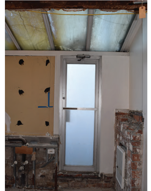
NORTH TERRACE DOOR, WINDOW & GLAZED ROOF LOWER LEVEL, LOOKING NORTH
