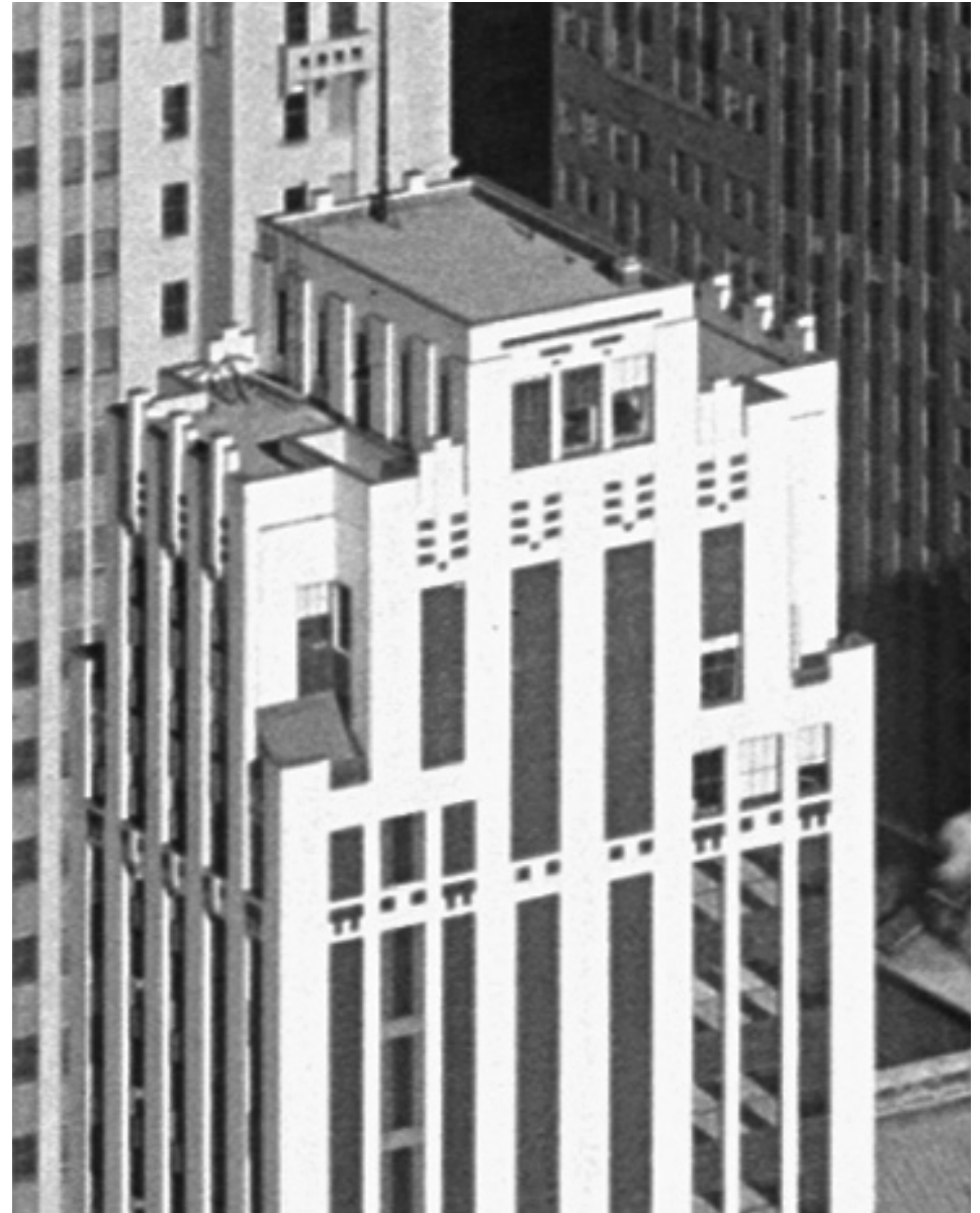
DETAIL - LOOKING NORTHEAST AT SOUTH ELEVATION Original Condition of Roof (Library of Congress)
