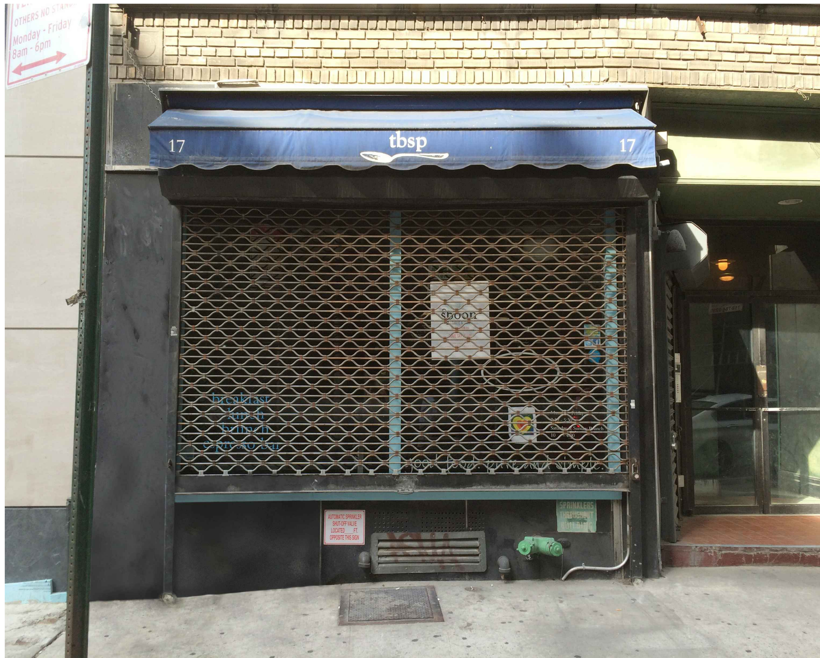
① EXISTING STOREFRONT - 08/31/2018
