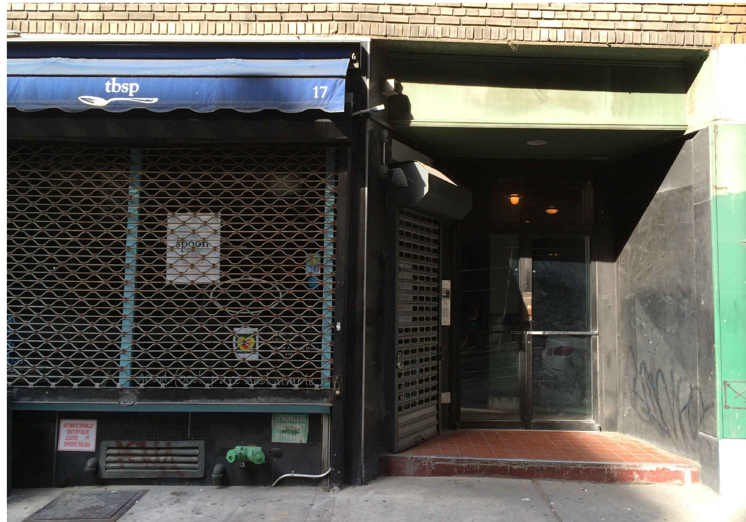
2 PREVIOUSLY EXISTING STOREFRONT - 08/31/2018
