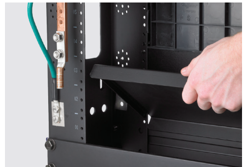
Bonding and grounding ready
