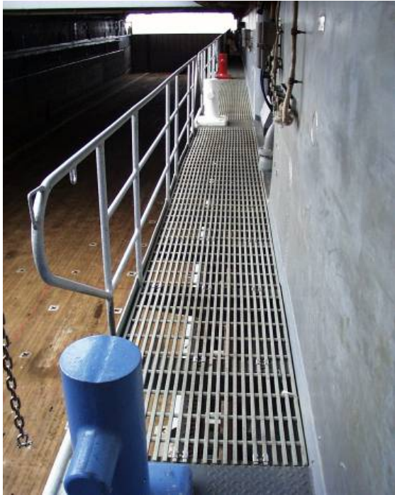
LSD Wing Wall
