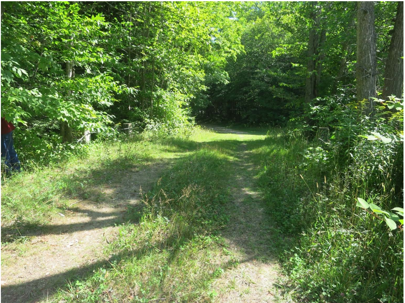
12. View east of the road crossing at the bridge, with concrete and cable railings shown, August 2022.
