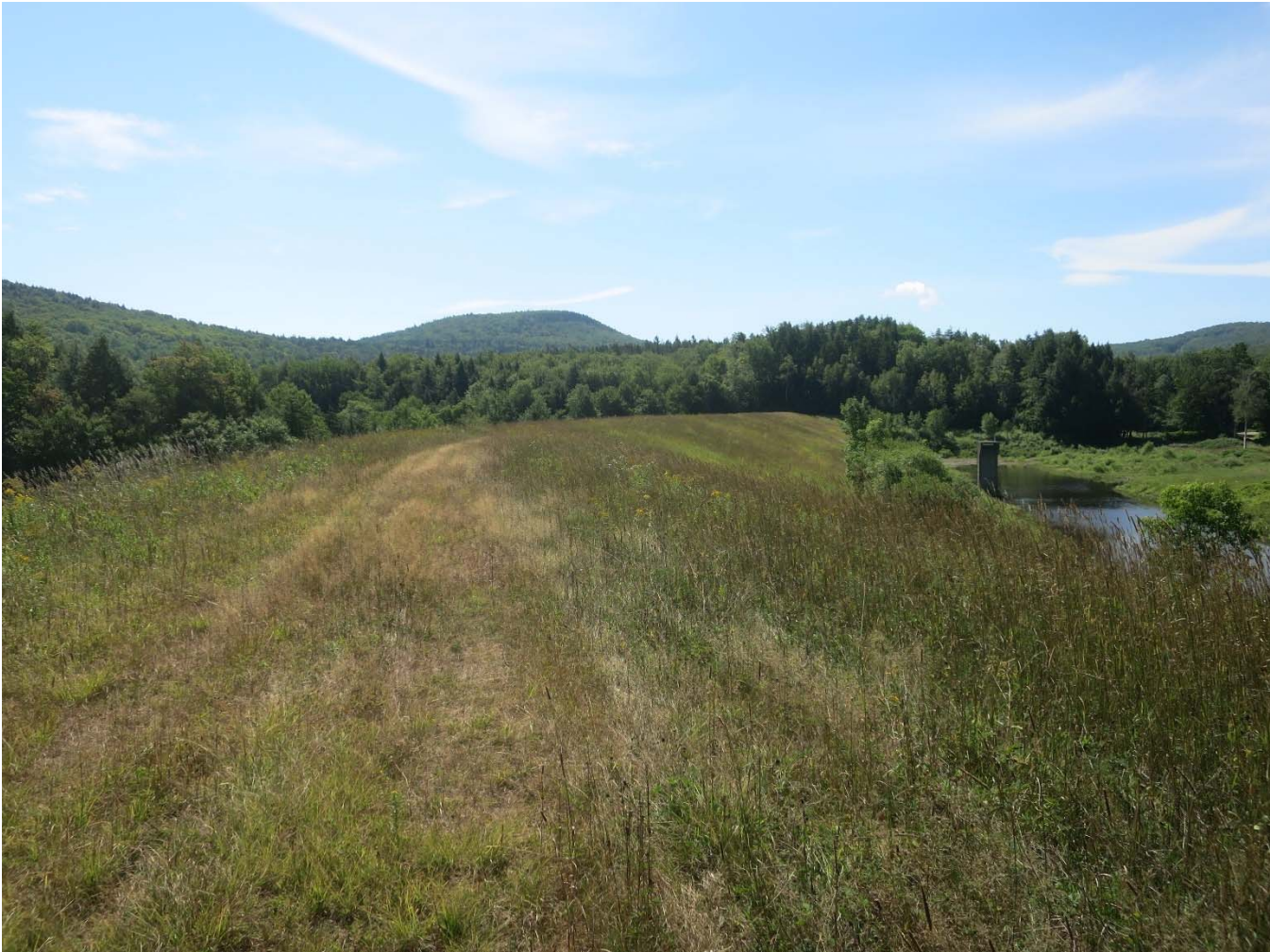
7. View south-southeast of the earthen dam at Site 2, with reservoir and intake at right, August 2022.
