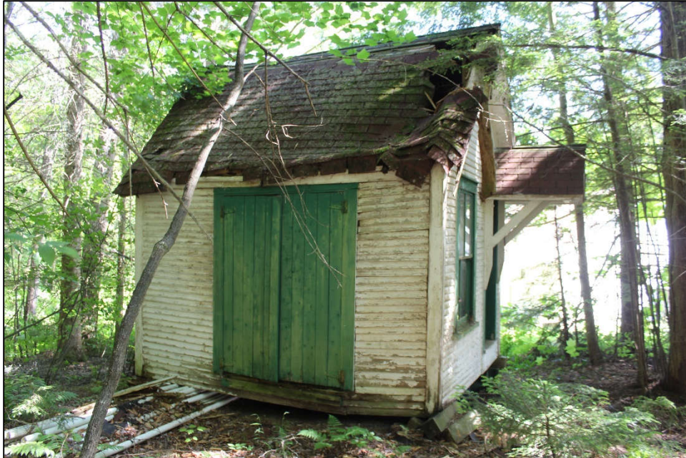
Photo 2. Dam 2, former water treatment building moved from its original location and used for storage, outside of the project APE. View to the northeast.
