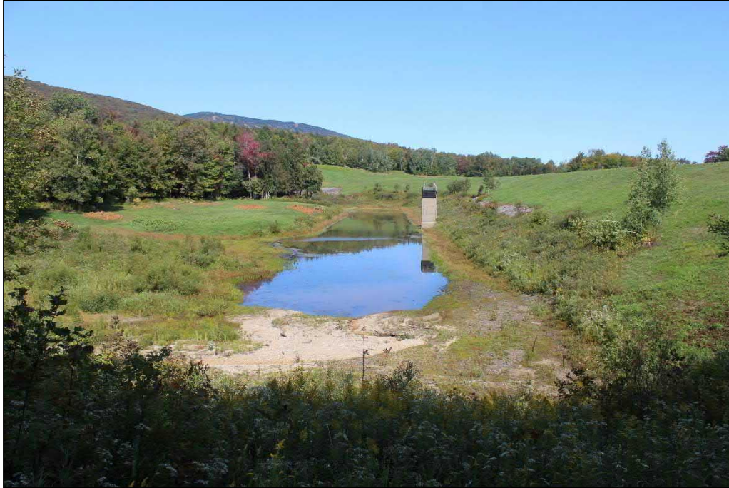
Photo 3. Site 2, overview of reservoir and dam to the right. View to the north.
