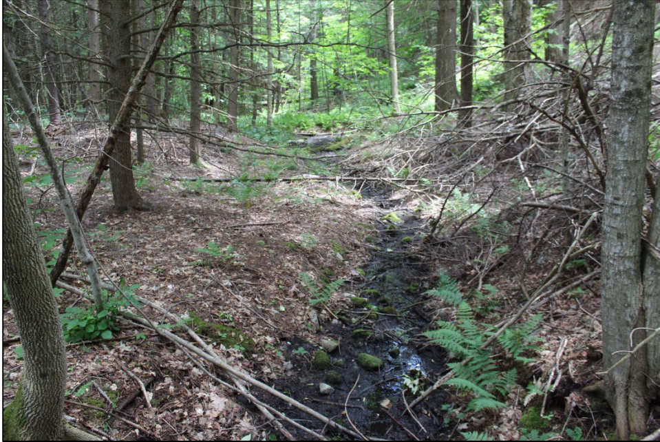
Photo 4. Dam 2, excavated ditch to direct surface water toward the water treatment facility, outside of project APE. View to the east.
