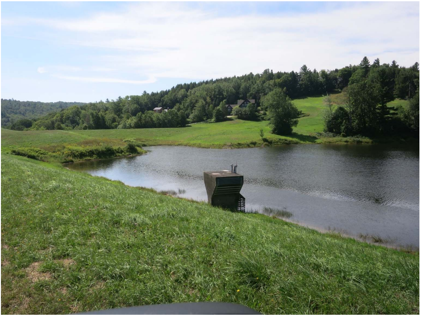
14. View south-southeast from top of earthen dam, showing intake structure at center and nearby dwellings, in the background, August 2022.
