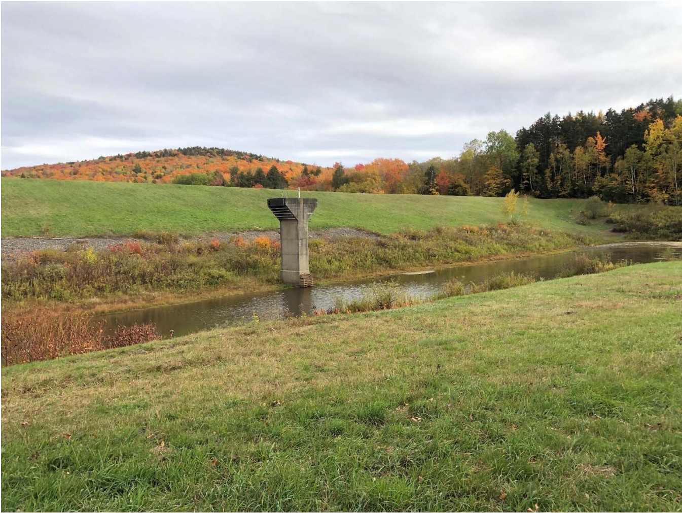
9. View of the reservoir with intake structure at center, October 2019.
