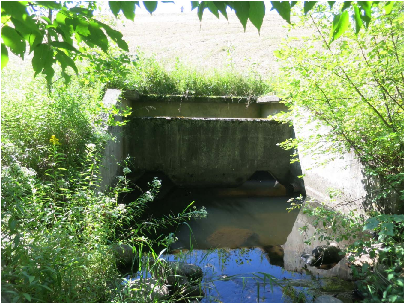
6. View south, showing the stilling basin and outlet structure, August 2022.
