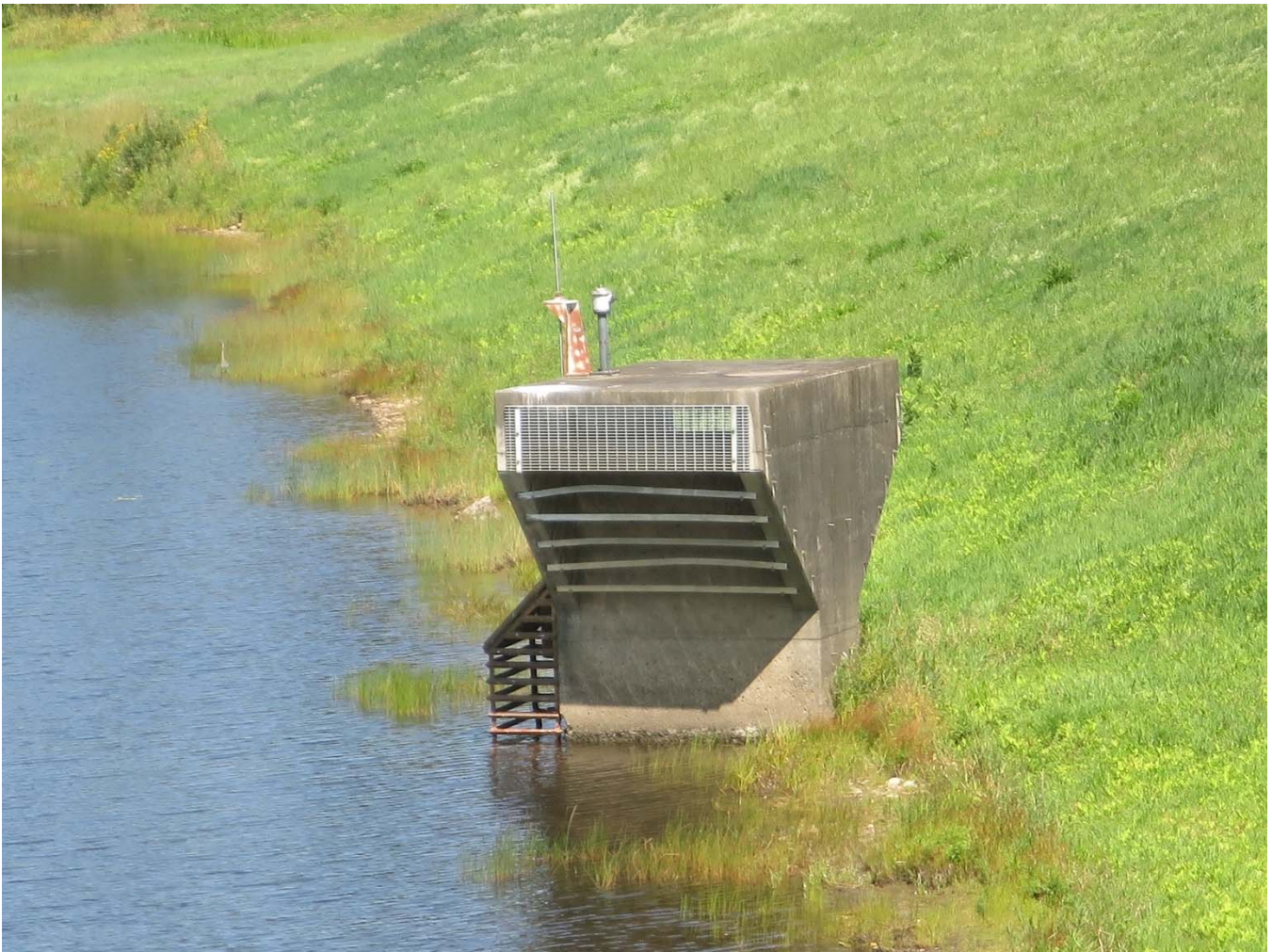
15. View north-northwest, showing intake structure, August 2022.
