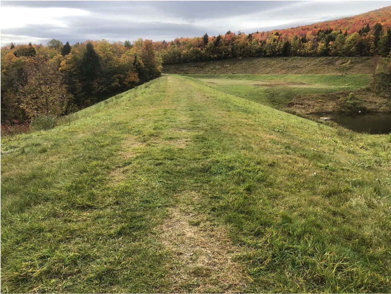
23. View south-southwest from the top of the earthen dam, October 2019.
