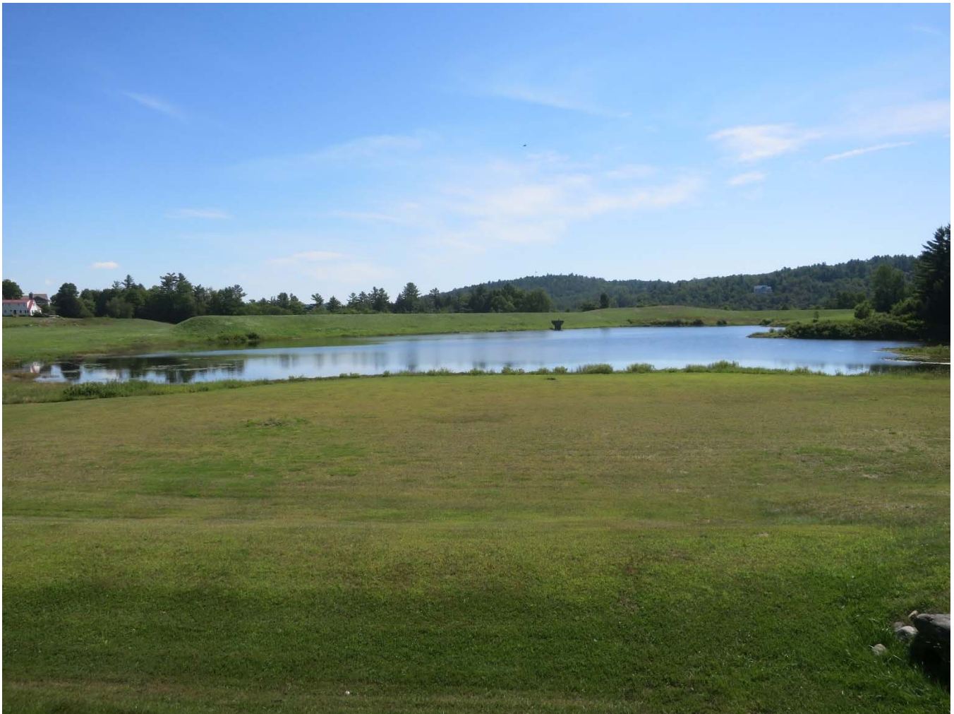
13. View east-southeast of Site 3, showing reservoir and earthen dam, in the background, August 2022.
