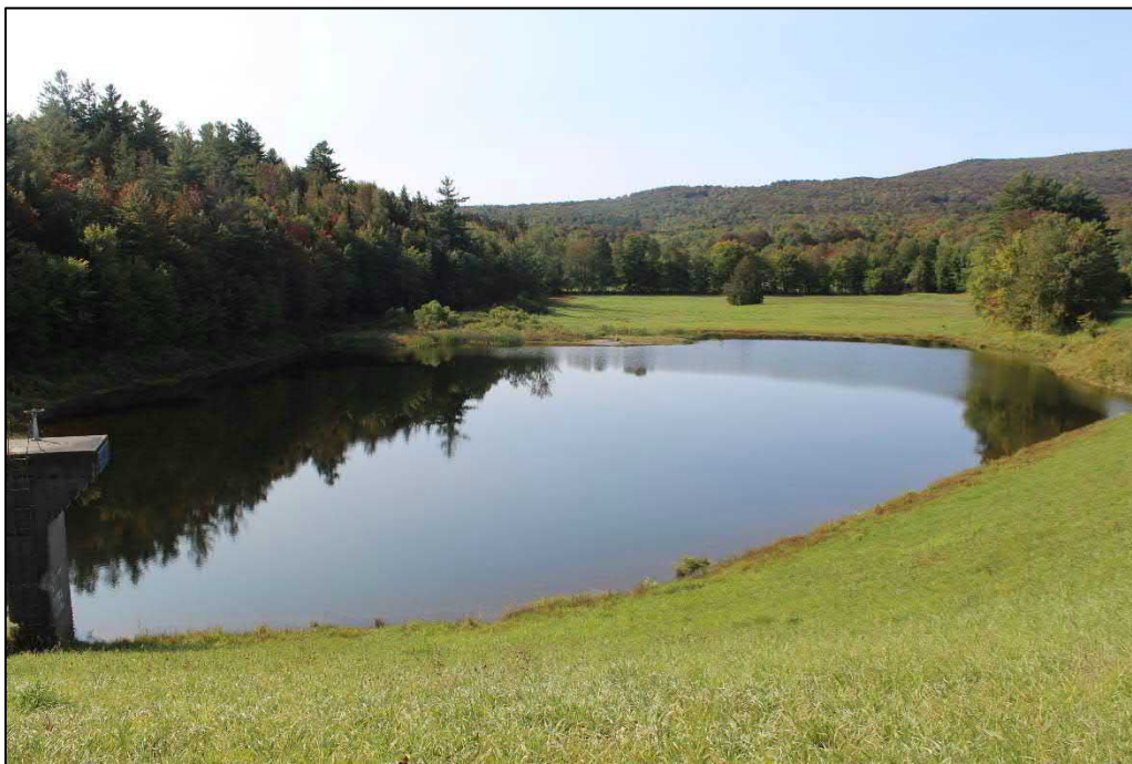
Photo 2. Site 1, existing reservoir in area of the farmstead and schoolhouse. View to the south.
