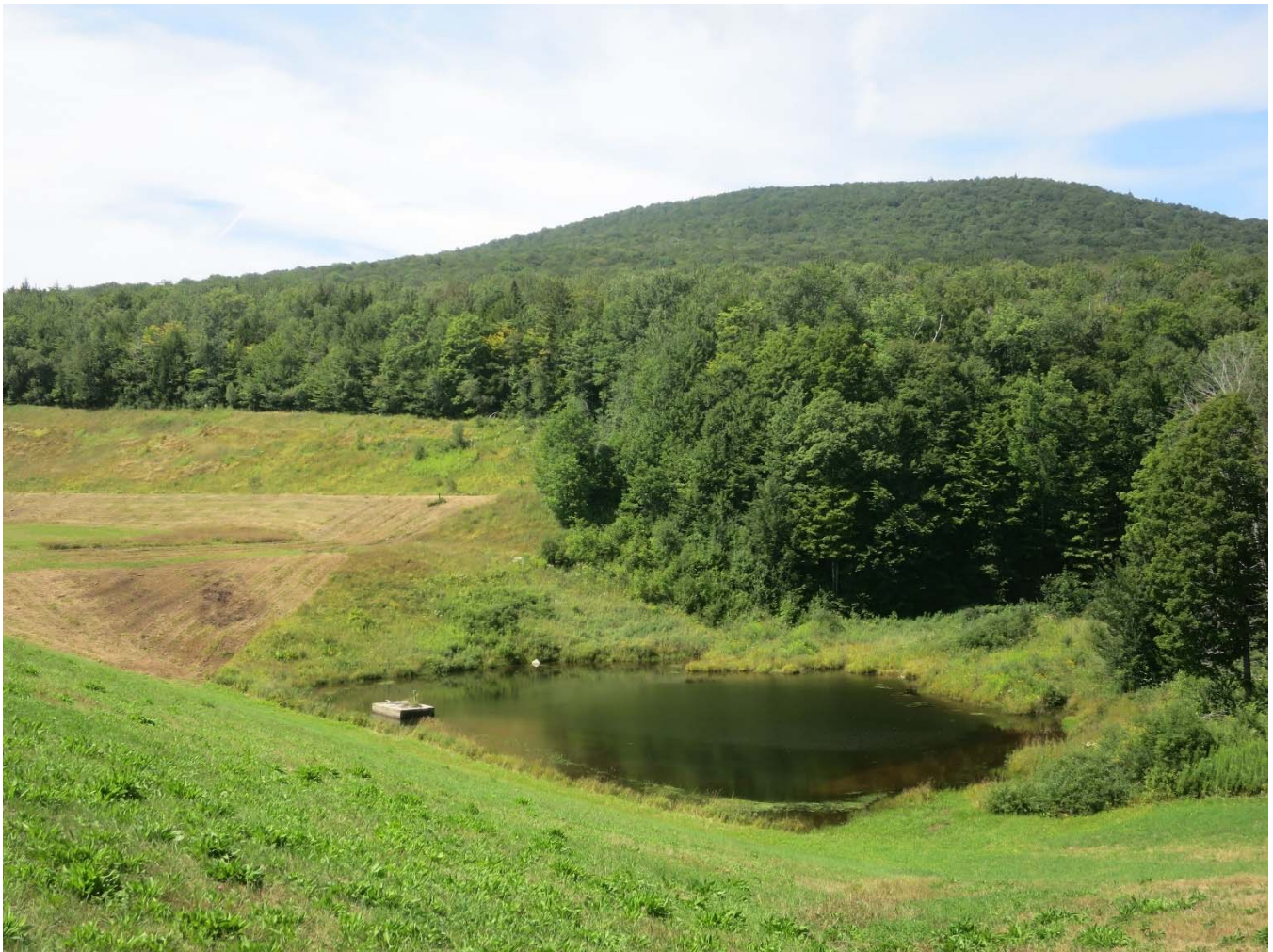
22. View west from the top of the dam, showing the reservoir, with embankment in background, August 2022.
