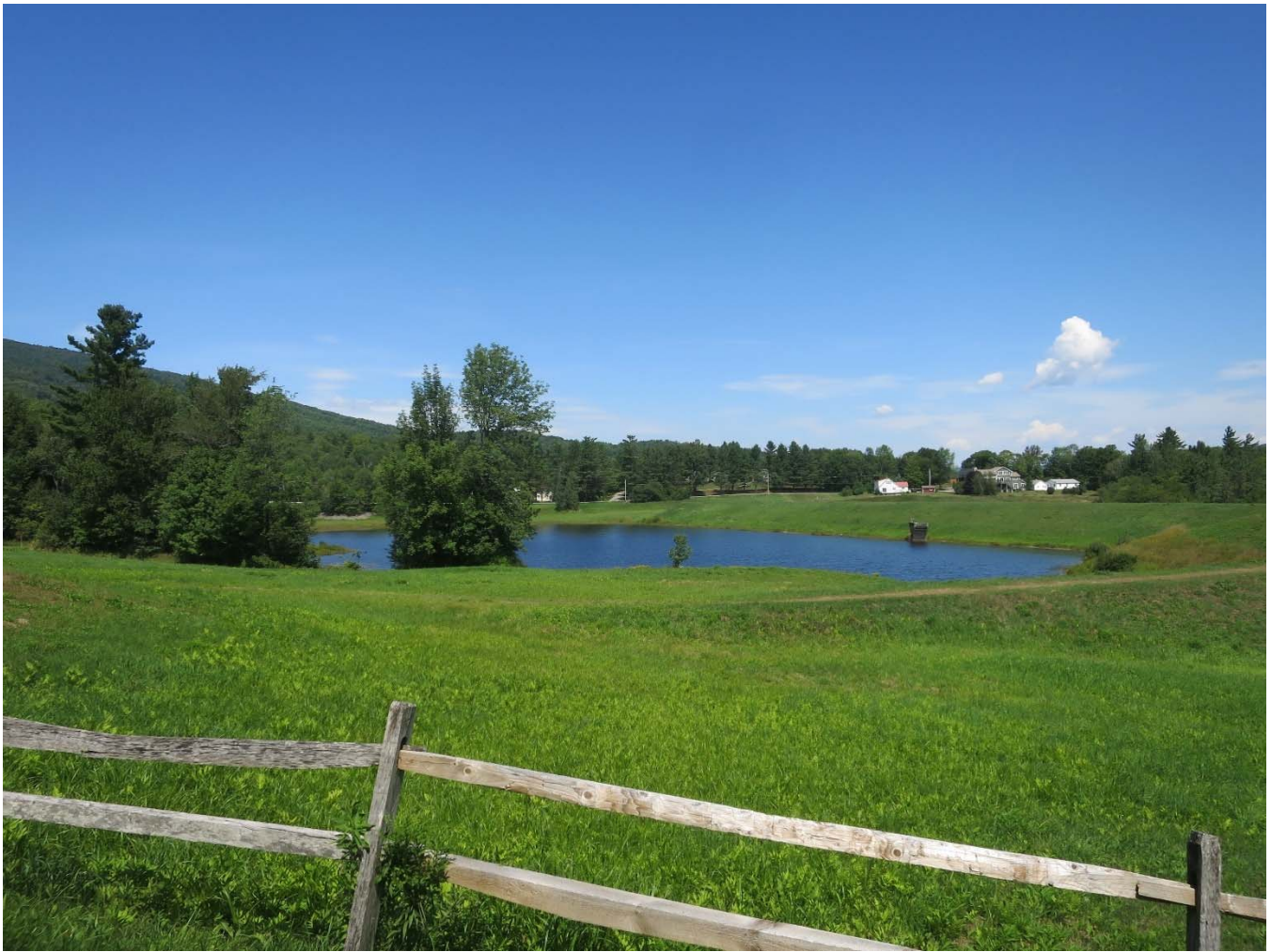
17. View north from a nearby private road, looking toward the reservoir and earthen dam, August 2022.
