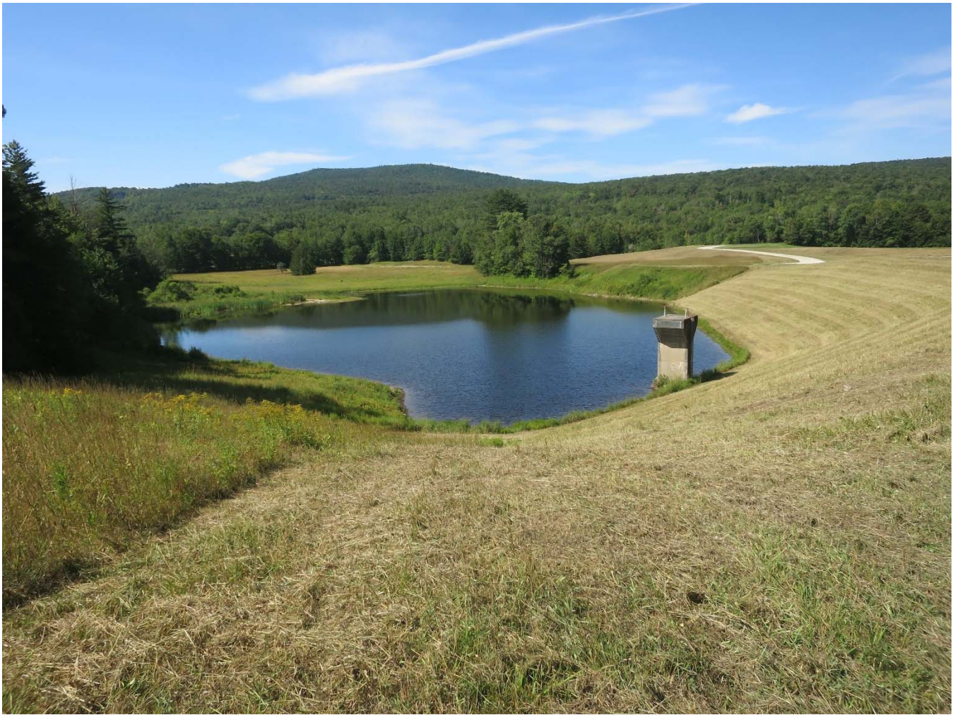
2. View west, showing reservoir and the intake structure, August 2022.
