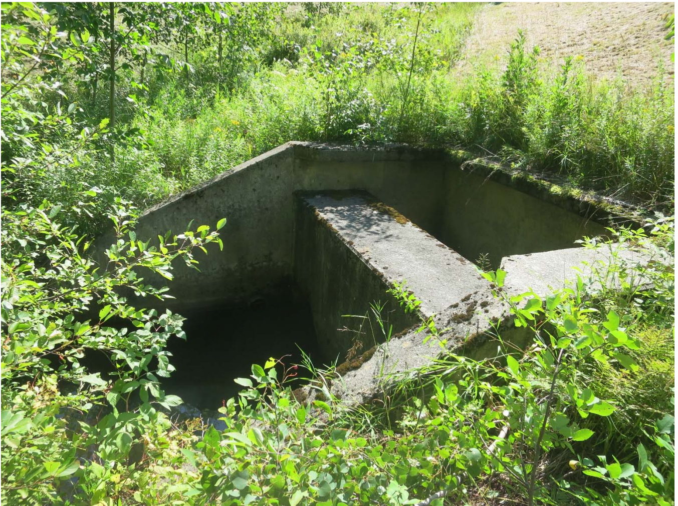
5. View southeast, showing the stilling basin and outlet, August 2022.
