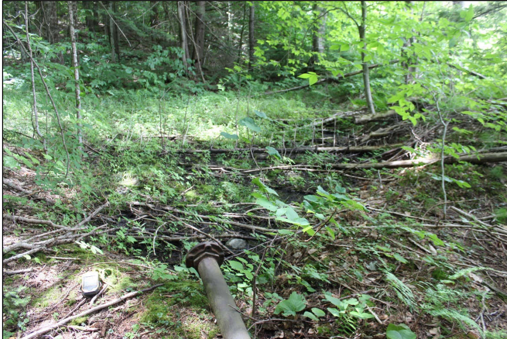
Photo 8. Dam 2, western pipe alignment end at small, excavated reservoir in the southwest corner of ASA 3. View to the southwest.
