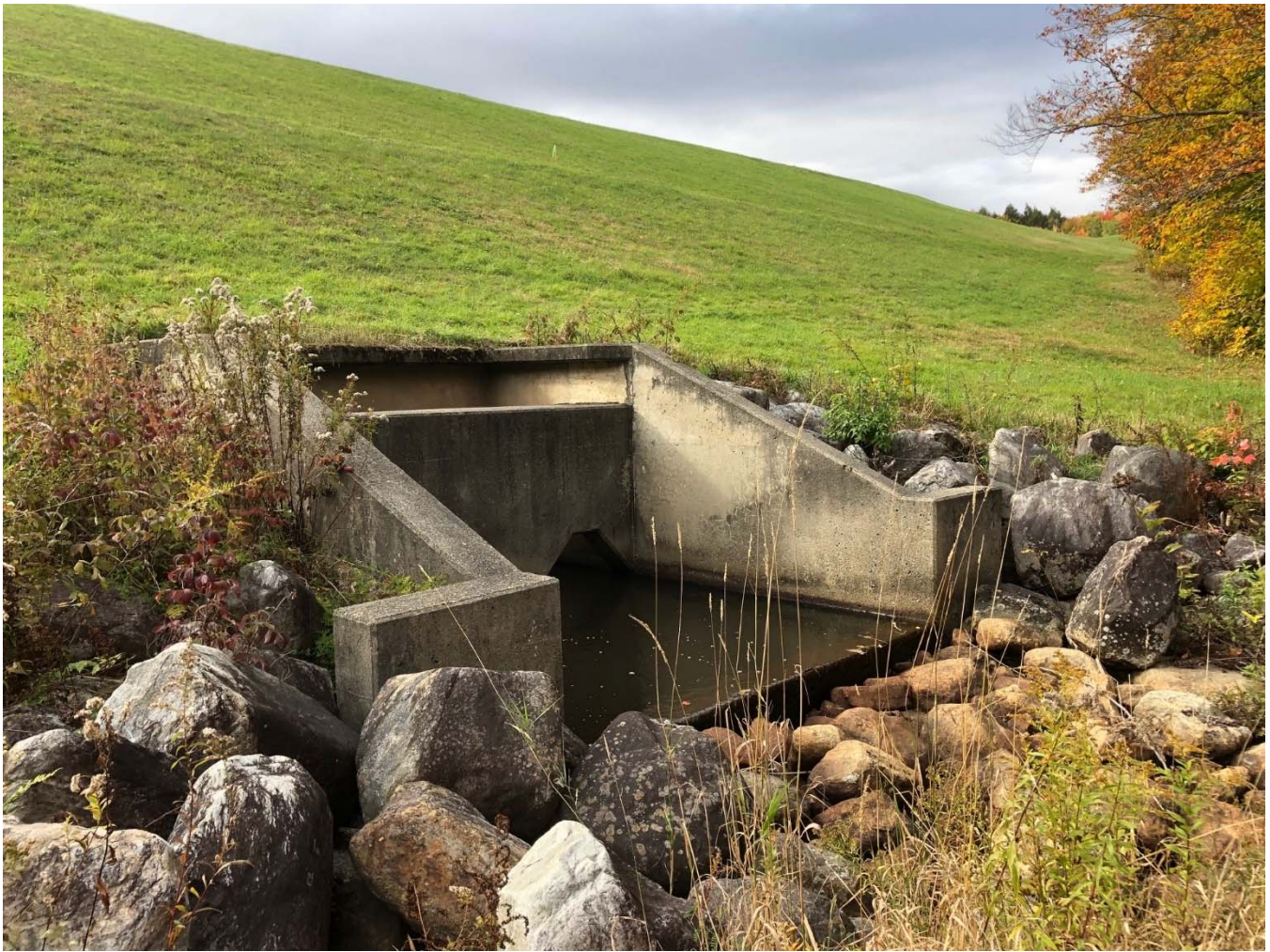
10. View of the stilling basin and outlet structure, looking west, October 2019.
