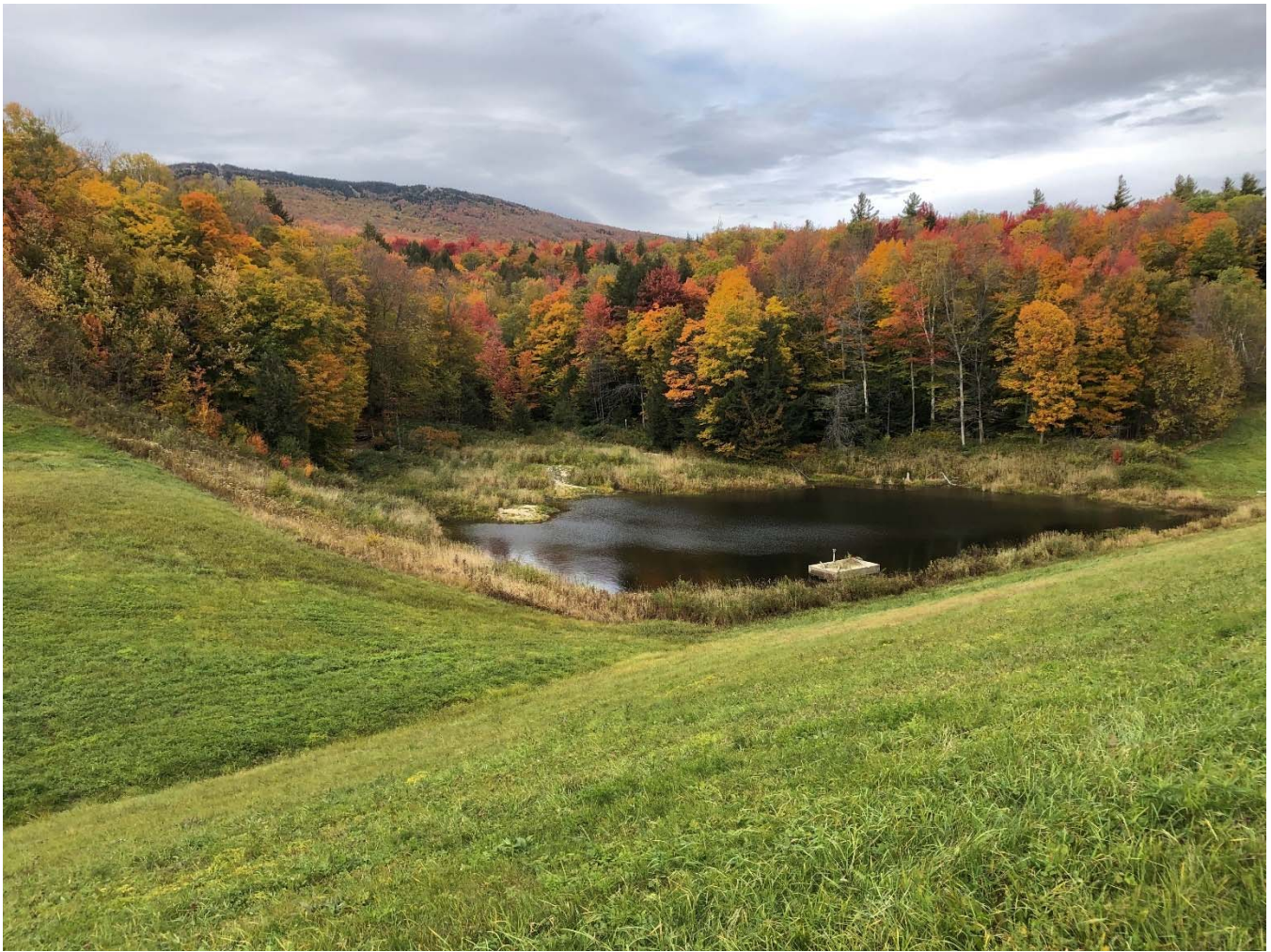
21. View north from the earthen dam, showing the reservoir with intake structure, at center right, October 2019.
