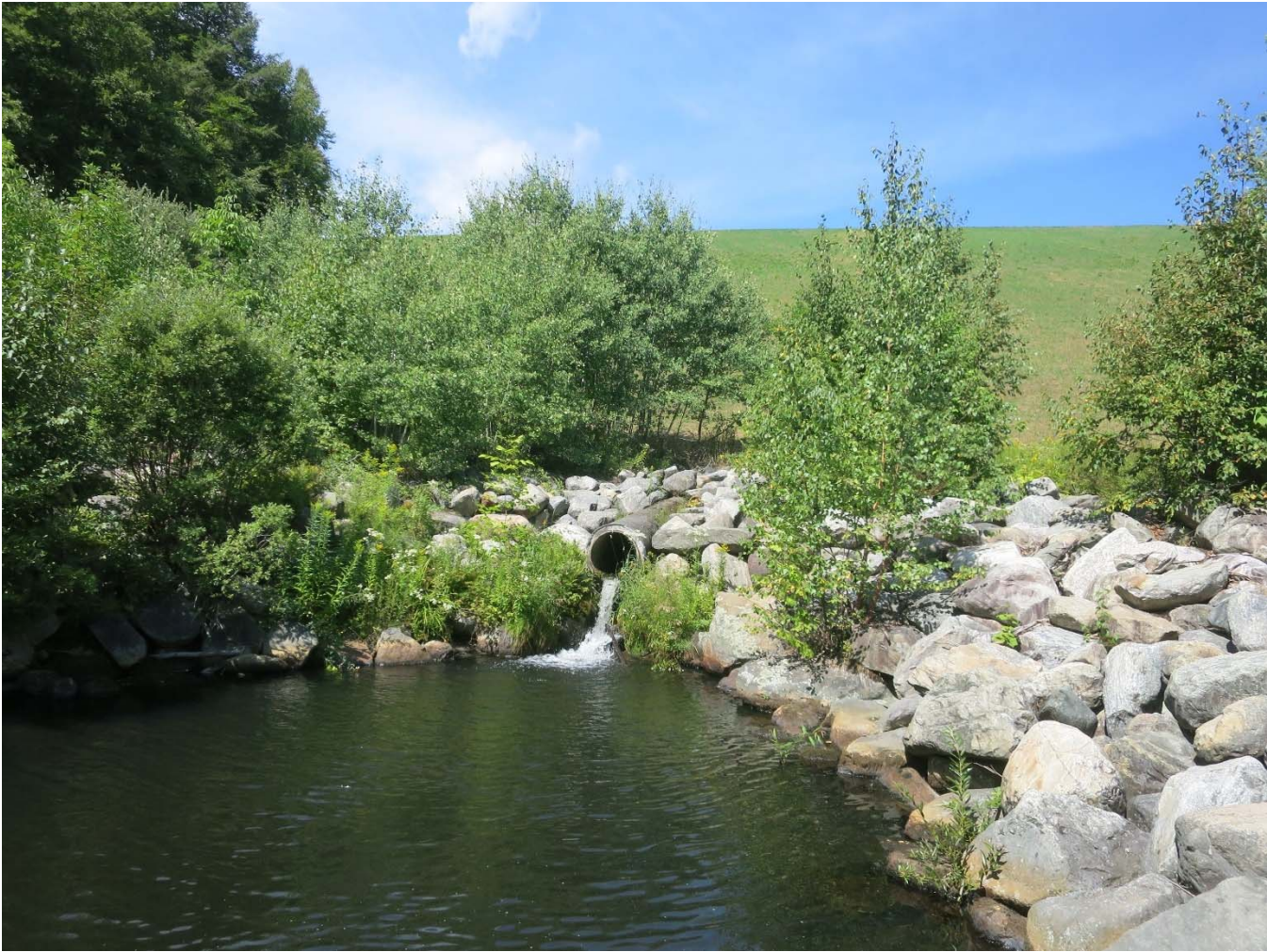
25. View west-northwest, showing the concrete outlet pipe, August 2022.
