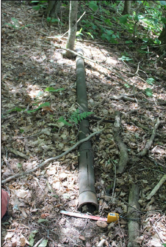
Photo 6. Dam 2, western pipe alignment between excavated reservoir and concrete wall, in the west end of the APE. View to the south.
