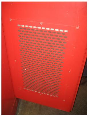
Figure F-7 Photo of open rounded-rectangular vent (LV switchgear)
