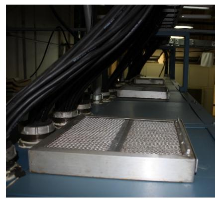
Figure F-4 External filter (shown on top of enclosure)
