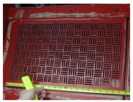
Figure F-6 Photo of open parquet vents (switchgear)
