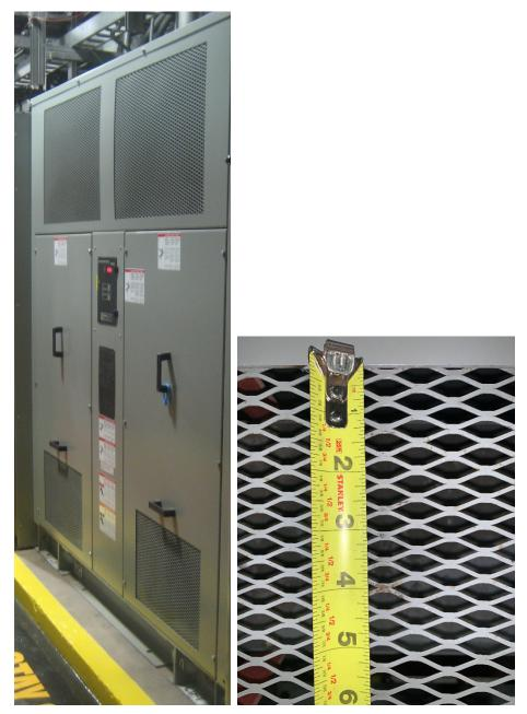
Figure F-9 Photo of expanded-metal vents on air-cooled transformer
