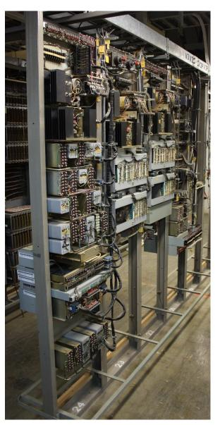
Figure F-11 Open-air instrumentation (not enclosed)
