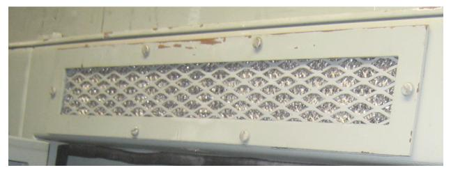
Figure F-3 Expanded metal vents with filters
