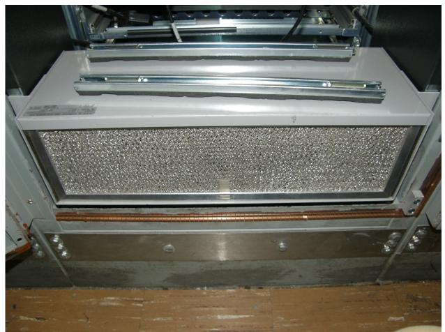
Figure F-2 Internal filter (shown with door open, filter surface area covers door vent area)
