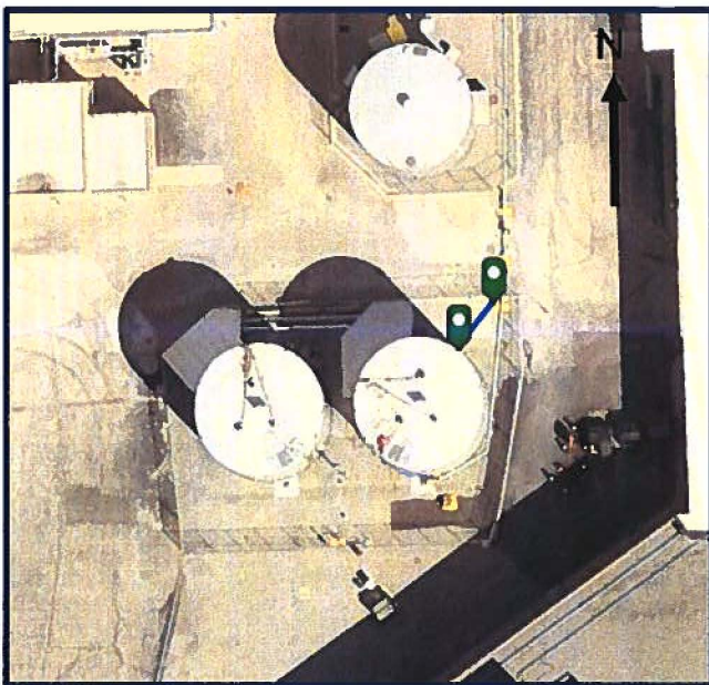
Figure 3: 2/3 Condensate Storage Tanks Resident
