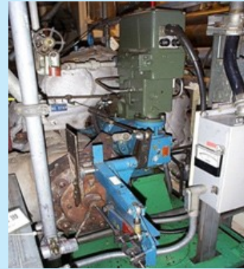
AFW pump trip and throttle valve
