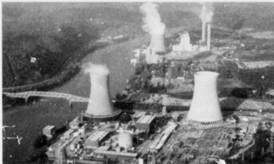
Construction of Beaver Valley Power Station Unit No. 2 (right) is approximately 59% complete. Duquesne Light owns 13.74 percent of Unit No. 2, which is scheduled to go on line in 1986. Like Unit No. 1 (left), Unit No. 2 is jointly owned by members of the Central Area Power Coordination (CAPCO) group but is being constructed and will be operated by Duquesne Light. For more information on CAPCO, see the inside back cover of this report.
