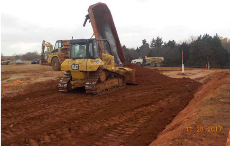
Photo 7: Backfilling GWI-UP1-01 with native material
