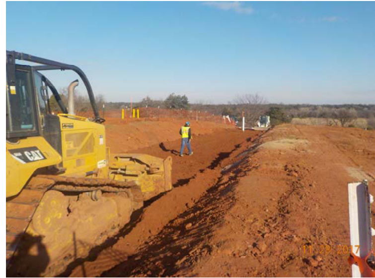
Photo 10: Backfilling GWI-UP1-02 with native material
