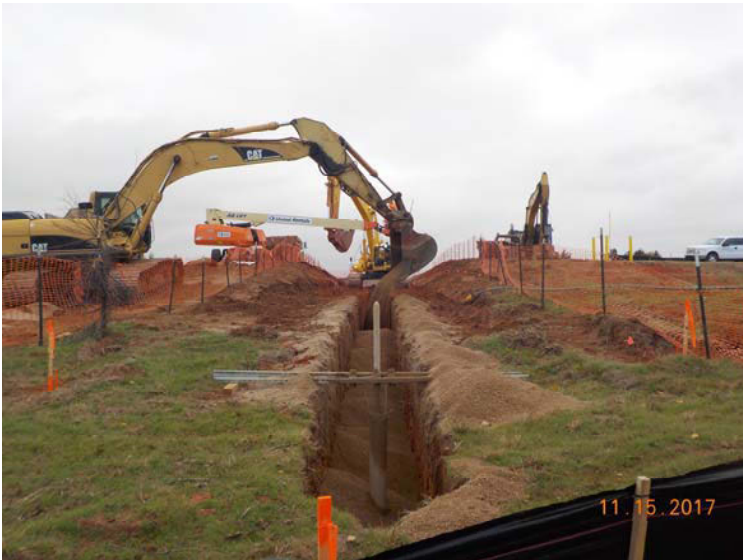
Photo 7: Backfilling with trench gravel and excavating GWI-UP1-02
