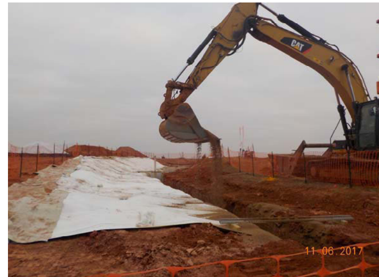
Photo 8: Backfilling GWI-UP2-01 with trench gravel
