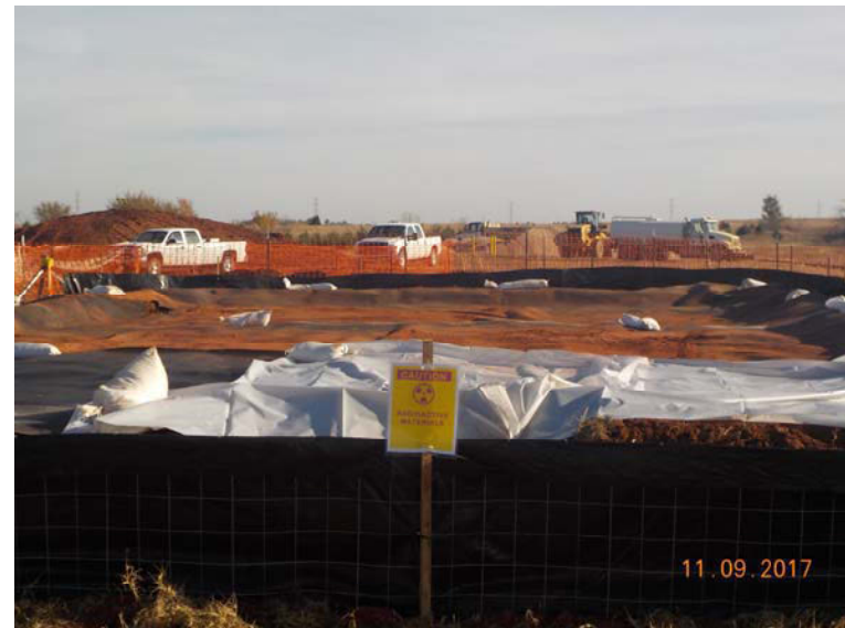
Photo 4: Staging area for potentially impacted materials
