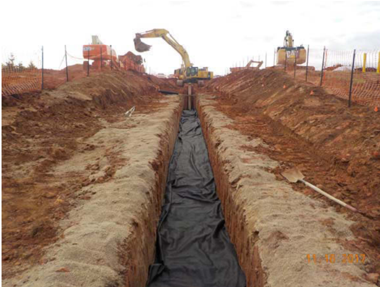
Photo 9: Placing geotextile in GWI-UP1-02
