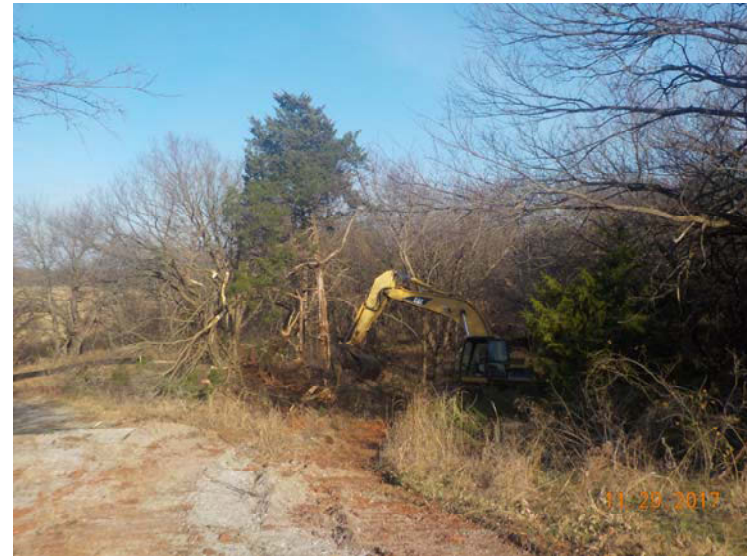
Photo 2: Clearing and grubbing
