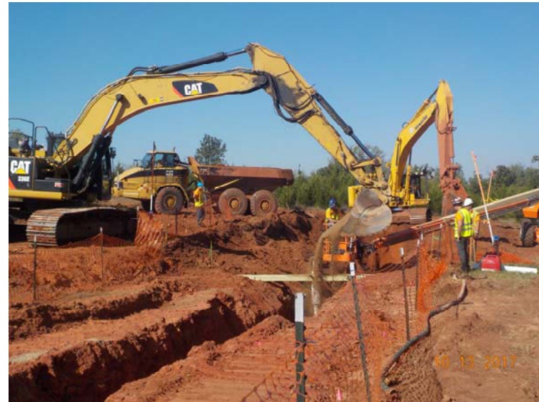
Photo 2: Backfilling GWI-BA1-01 with trench gravel
