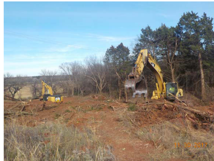
Photo 4: Clearing and grubbing
