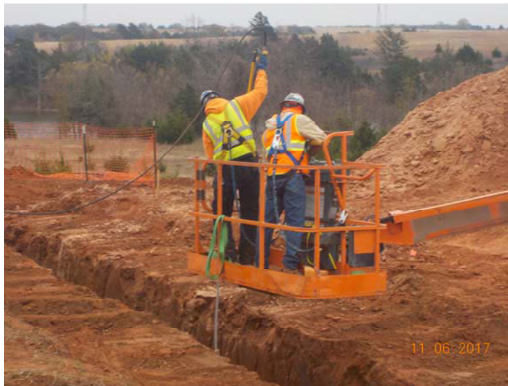
Photo 7: Pressure washing the north wall of GWI-UP2-01 from Station 4+00 to Station 4+75
