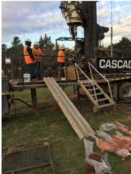
Photo 3: Monitor well installation
