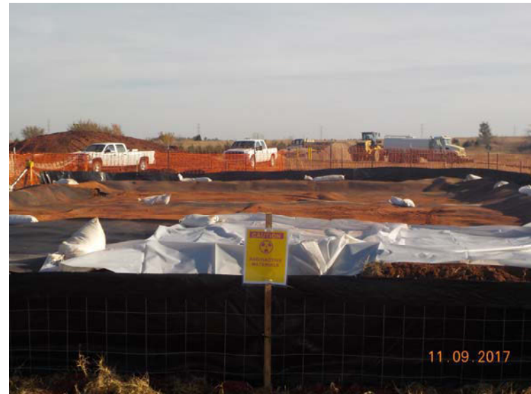
Photo 4: Staging area for potentially impacted materials
