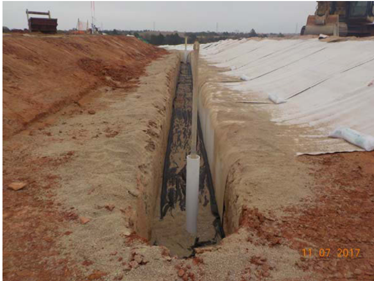
Photo 5: Placing geotextile in GWI-UP2-01
