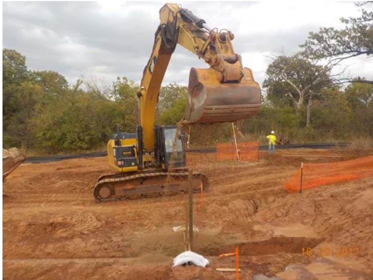
Photo 5: Backfilling GETR-BA1-01 with trench gravel
