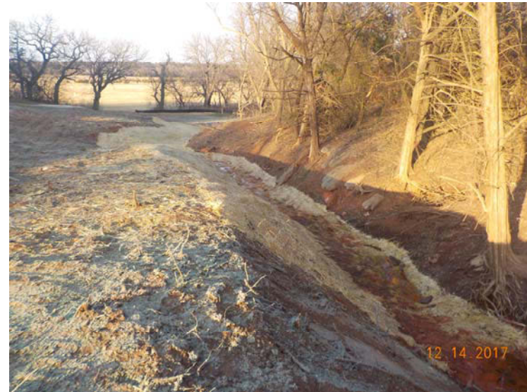
Photo 6: Seed and erosion control mats
