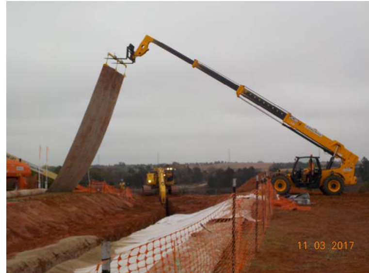
Photo 6: Installing Geosynthetic Clay Liner on the south wall of GWI-UP2-01
