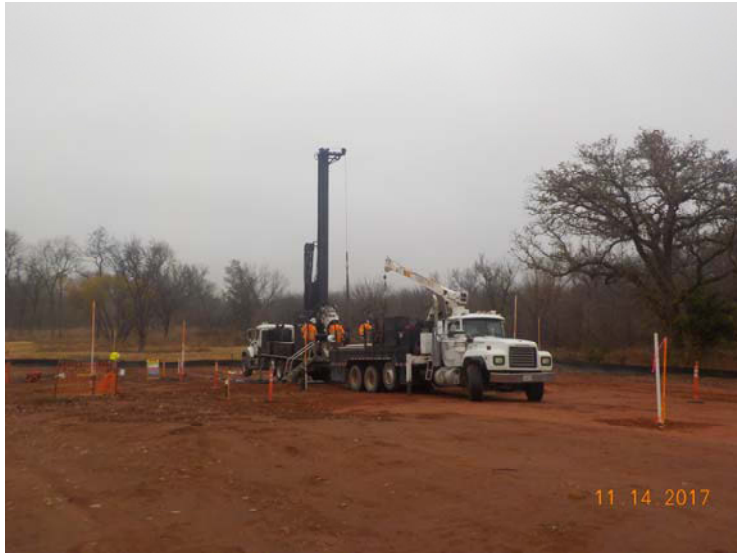
Photo 1: Monitor well installation
