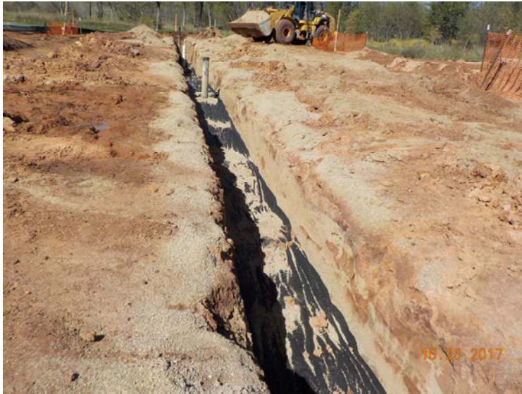
Photo 5: Placing geotextile in GETR-BA1-01
