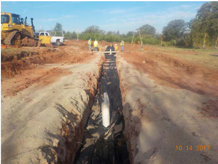
Photo 7: Placing geotextile in GWI-BA1-01
