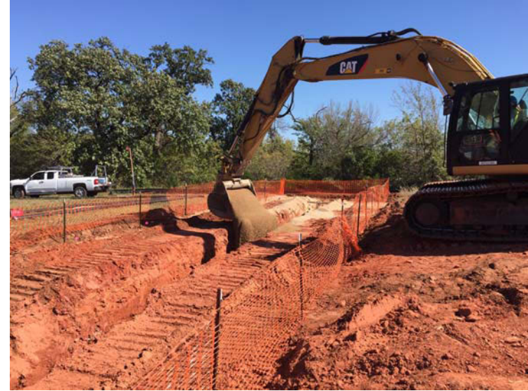
Photo 6: Backfilling GWI-BA1-01 with trench gravel
