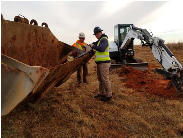
Photo 3: Enercon scanning equipment and removed monitor well for radiological activity
