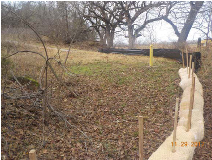
Photo 1: SWPPP BMP installation
