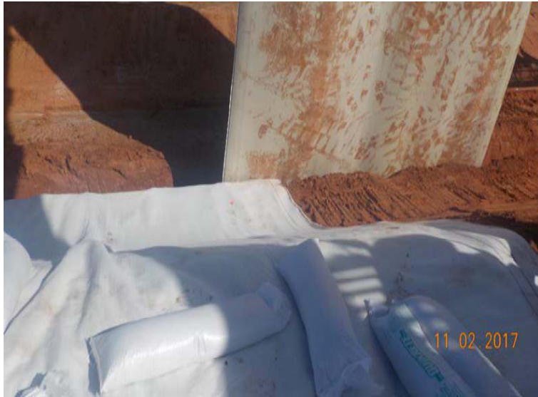
Photo 5: Installing Geosynthetic Clay Liner on the south wall of GWI-UP2-01
