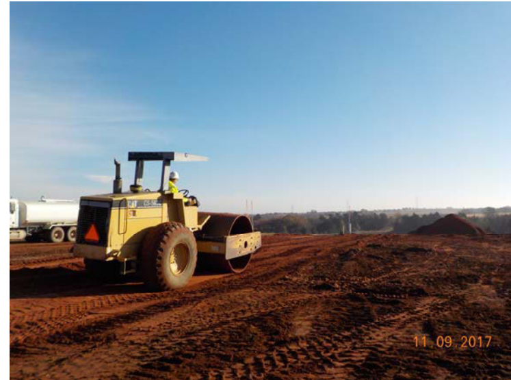
Photo 6: Backfilling GWI-UP2-01 with native material
