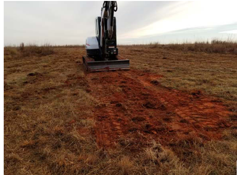
Photo 4: Area backfilled after monitor well removal
