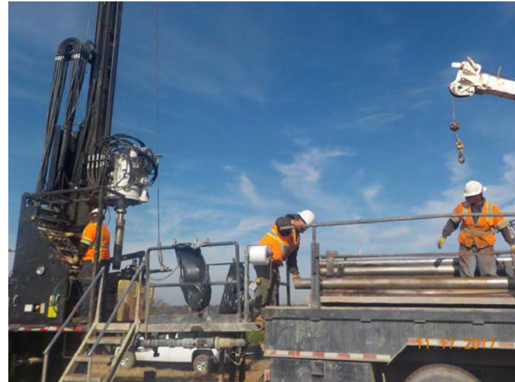
Photo 2: Monitor well installation
