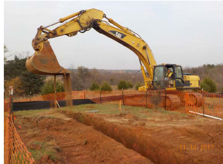
Photo 6: Backfilling GWI-UP1-02 with trench gravel
