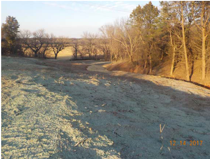
Photo 5: Seed and erosion control mats
