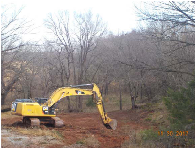
Photo 3: Clearing and grubbing
