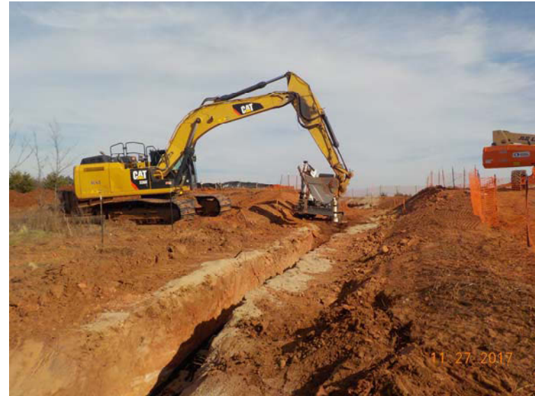
Photo 6: Backfilling GWI-UP1-01 with native material
