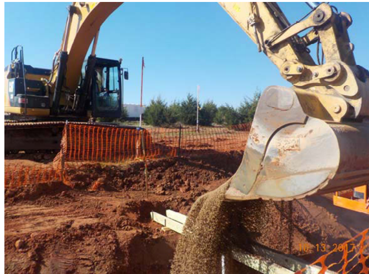
Photo 4: Backfilling GWI-BA1-01 with trench gravel
