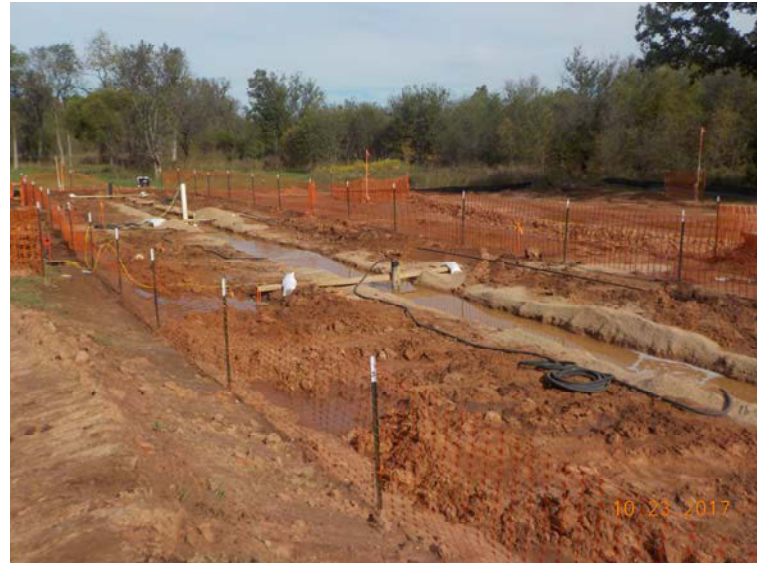
Photo 8: Circulating slurry breaking agent in GETR-BA1-01
