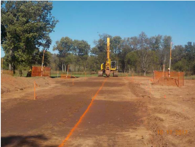
Photo 1: Working platform for GETR-BA1-01
