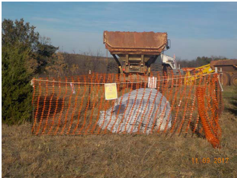
Photo 3: Concrete removed from GWI-UP1-02
