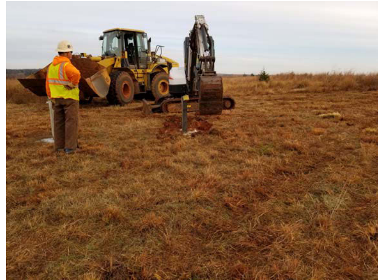
Photo 2: Removal of monitor well
