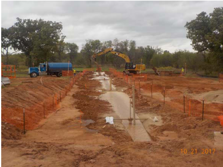
Photo 7: Backfilling GETR-BA1-01 with trench gravel transporting slurry to frac tanks
