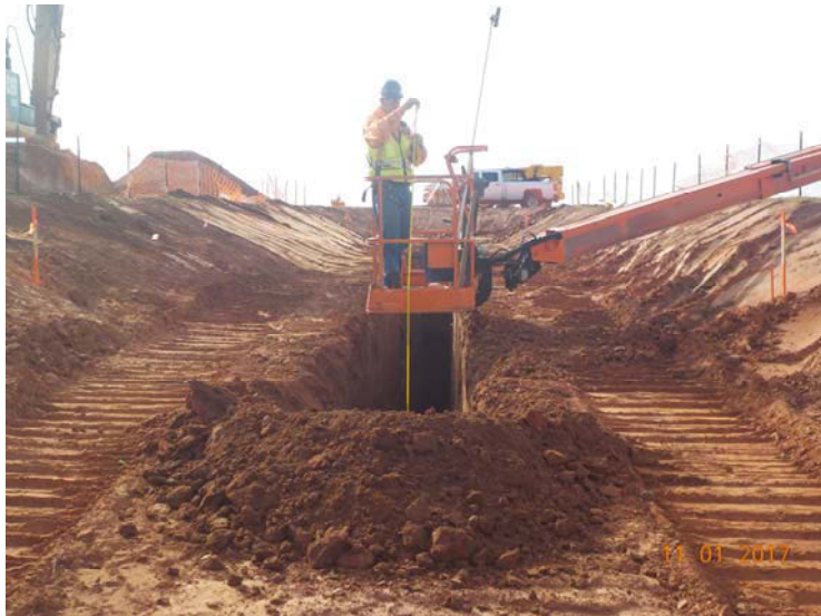
Photo 3: Confirming depth of GWI-UP2-01
