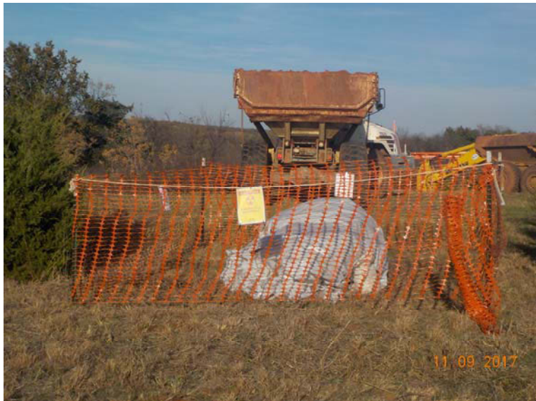
Photo 3: Concrete removed from GWI-UP1-02
