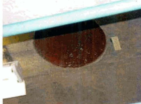
Photo 2, P141S1028 Bottom Side Room 1307 and Fire Area A-8
