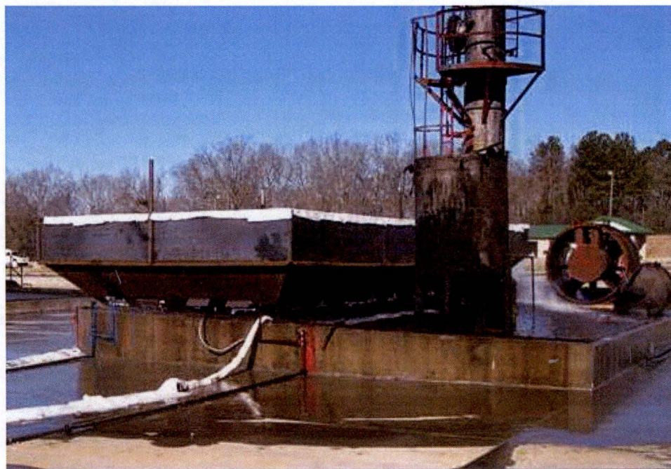
Viewed from Southwest – Other Structures Are Props Used for Firefighter Training
