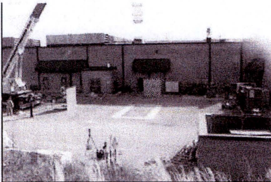
Figure 2.12.1-2 – CTU2 prior to drop
