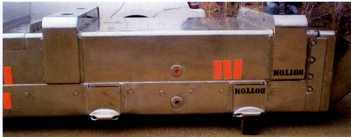
Figure 2-12 – Bottom End Stiffener Damage
