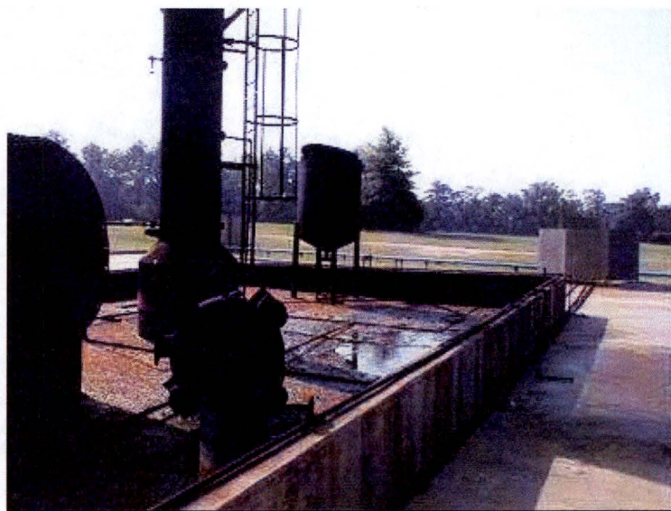
Viewed from Southwest – Other Structures Are Props Used for Firefighter Training
