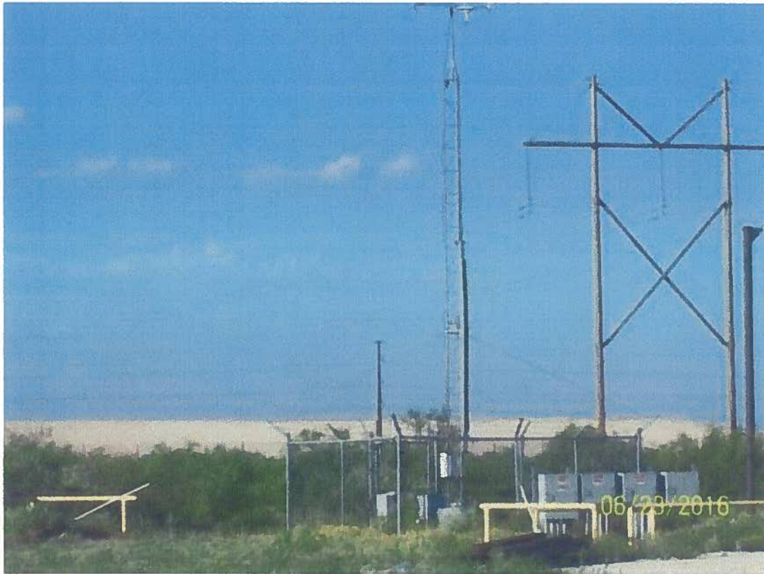
Figure 2-21 Tower 1 Located South of the WCS Guard House
