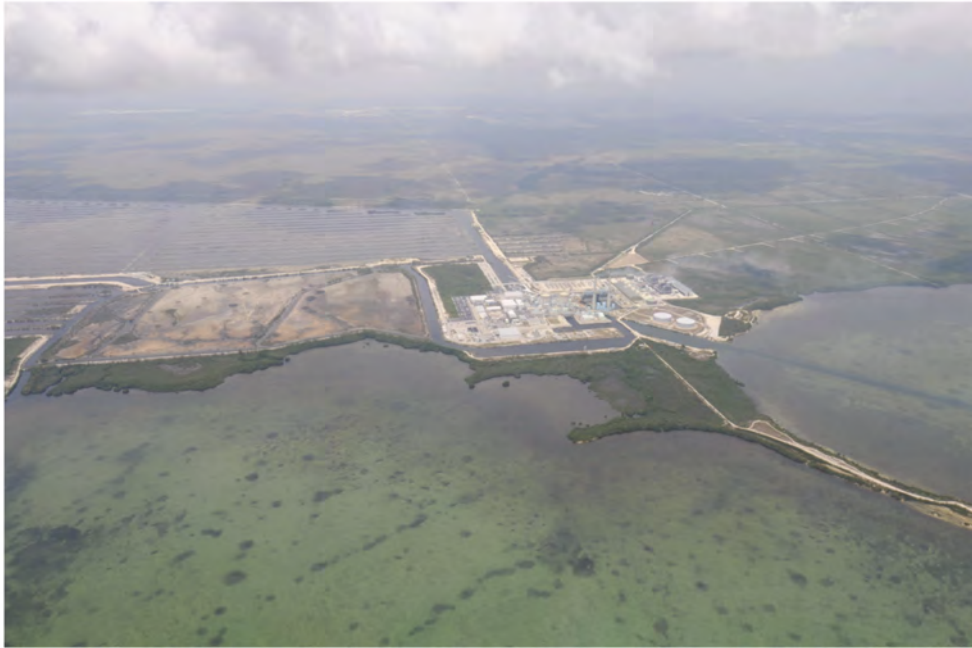
Looking west, Units 6 & 7 plant area shown to left, Units 1–5 shown to right
