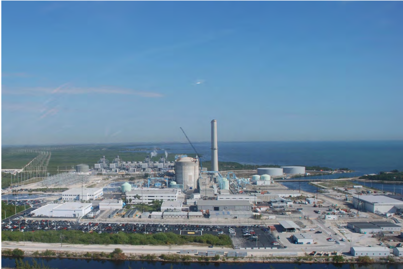
Figure 3.1-1 Existing Turkey Point Units 1 to 5
