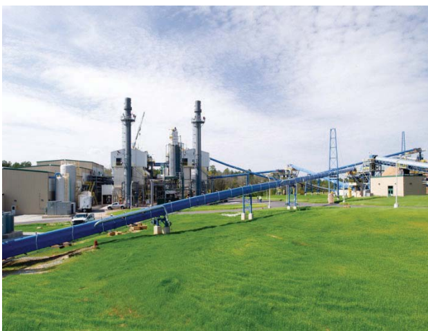
Figure 2-4 View of the Biomass Cogeneration Facility
