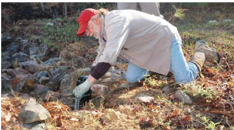
Figure 4-8 Installation of a Stormwater Sampling Device at an Industrial Stormwater Outfall
