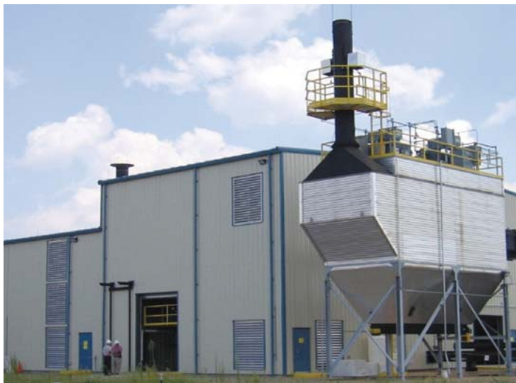
Figure 2-3 A-Area Biomass Steam Plant
