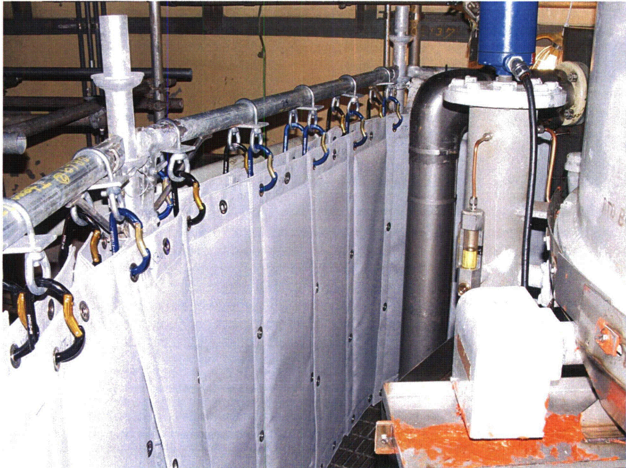
Figure 2: Lead Blanket Installed at Salem
