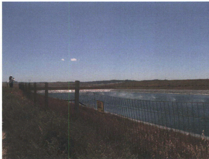
Figure 2: Northeast Corner of Pond 3
