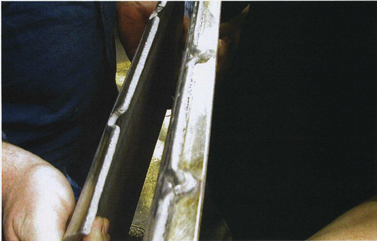
FIGURE 2.12.7-6 – Close-up View of TS-2 Failed Fillet Weld Joint
