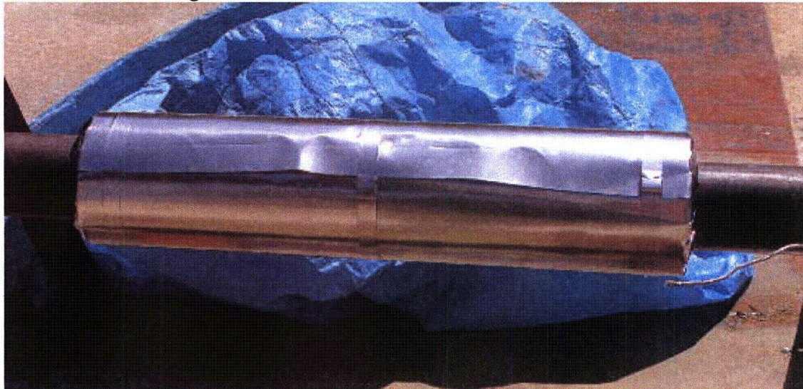
Figure 3b3-12 Jacketed Armaflex Insulation Test 3
