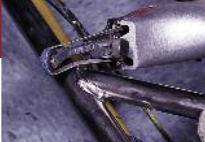
Blending a weld using a portable file belt.
