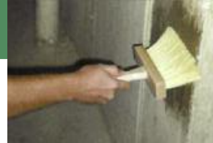
Applying waterproofing material with a masonry brush.
