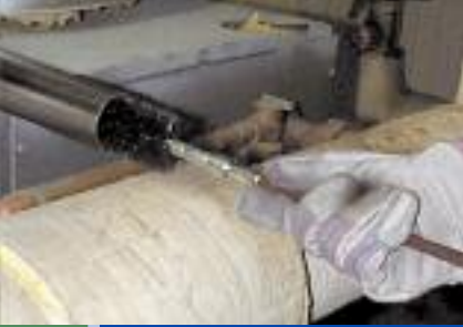
Cleaning boiler pipes with a flue brush.
