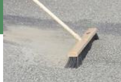
Sweeping cinders from the surface of a parking lot.
