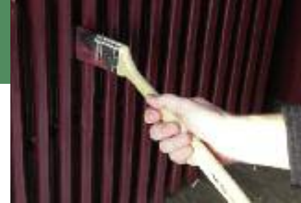
Painting inside the fins of a radiator with a Radiator brush.
