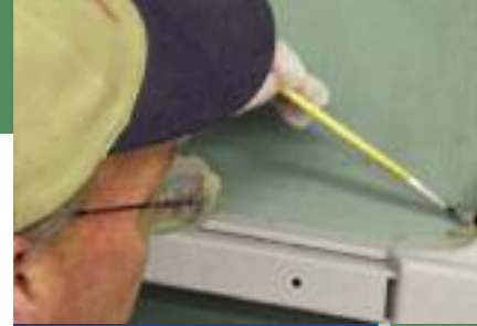
Painting a tight area on a steel door with a Marking Brush.
