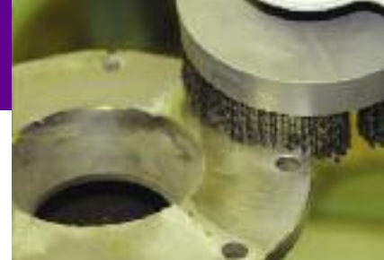
Removing gasket material from a pipe flange.
