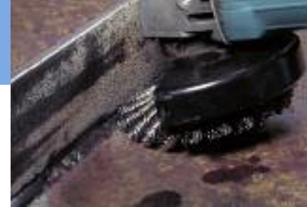
Cleaning a corner weld with a bevel brush.
