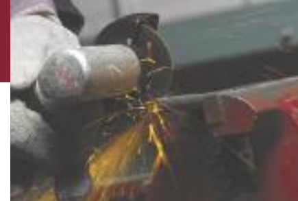
Cutting a piece of steel tubing to length.
