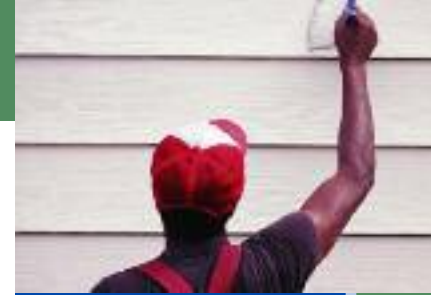
Applying paint to clap board siding.
