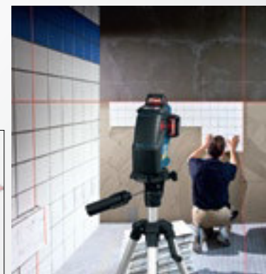
Level and Square to Install Tile
