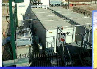
Frequency Changers (FC) DB Energie (Germany),11 units installed to date, 18 MVA each
