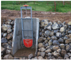
Remove existing manual gate and...
