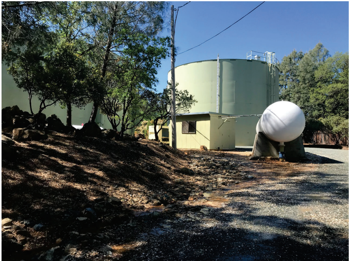
Existing pump station building, pressure tank, and storage tank from entrance, south view
