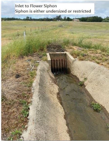
Lincoln Canal near Monment Pl Canal undersized
