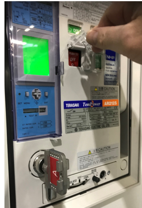
Figure 1 Key in OFF, ACB OFF button retracted
