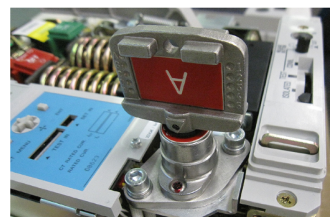
Figure 3 Allen-Bradley ProSafe trapped key lock fitted with the ACB cover removed
