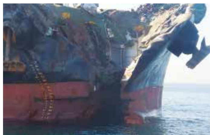
The damaged bow of the tanker Alexandra 1 following the collision with the UK-flagged containership Ever Smart . Picture: MAIB
