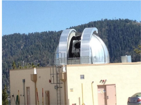
Figure 11.34: JPL's OCTL showing a 1-meter optical aperture. Credit: NASA JPL.
