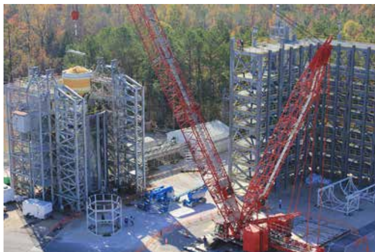
The Integrated Structural Test at Marshall included applying loads 40 percent greater than expected during launch to test versions of the launch vehicle stage adapter, frangible joint assembly, ICPS, Orion stage adapter, and a mass simulator for Orion.
