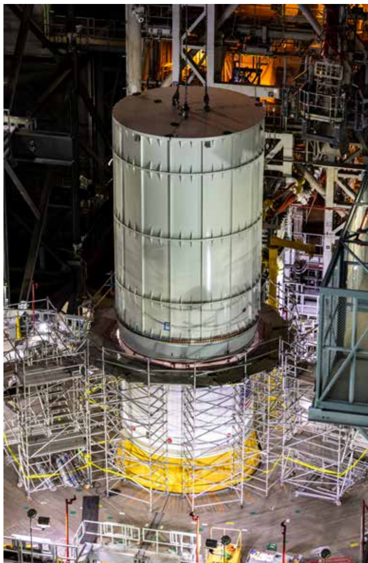
Modal testing underway in High Bay 3 inside the Vehicle Assembly Building at Kennedy, using the Orion stage adapter structural test article and the mass simulator for Orion. The test hardware articles have the same weight and mass characteristics as their respective flight components.
