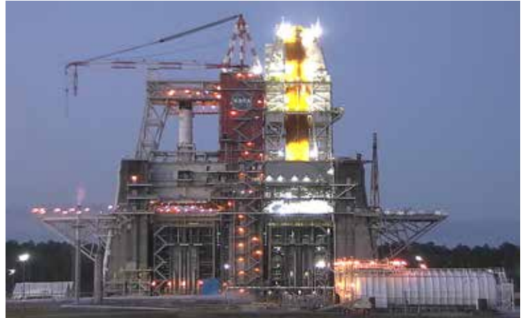
NASA Stennis provides unique facilities for testing SLS RS-25 engines and controllers.
