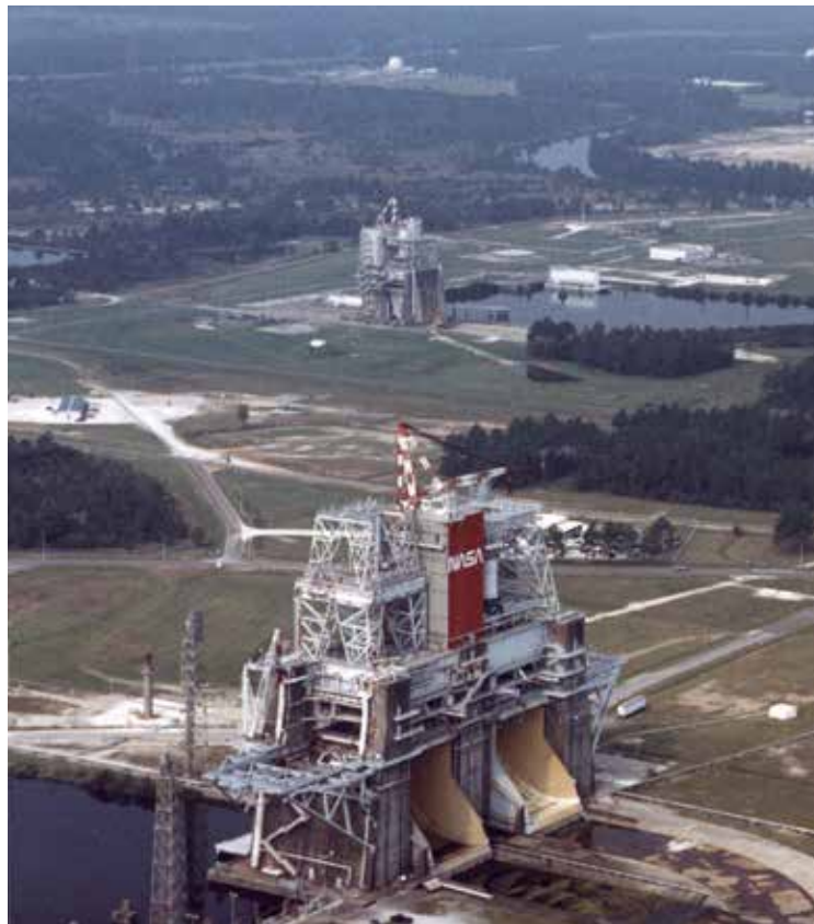
NASA Stennis provides unique facilities for testing SLS RS-25 engines and controllers. The B Complex, foreground, was used for Green Run testing the SLS core stage.
