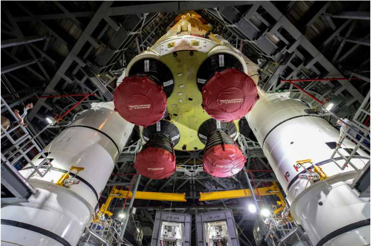
The Artemis I core stage is lowered between the SLS solid rocket boosters in the Vehicle Assembly Building. The SLS design uses a proven propulsion system of solid rocket boosters and liquid-fuel RS-25 engines to launch more payload to the Moon than any rocket since the Saturn V.
