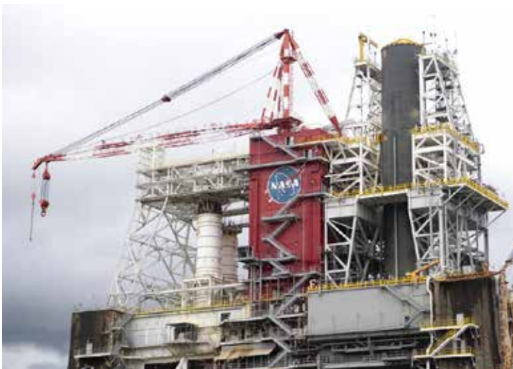
A full-scale SLS core stage pathfinder was used by crews at Michoud, Stennis, and Kennedy to practice handling, logistics, crane lifts, and other operations before working with Artemis I flight hardware.
