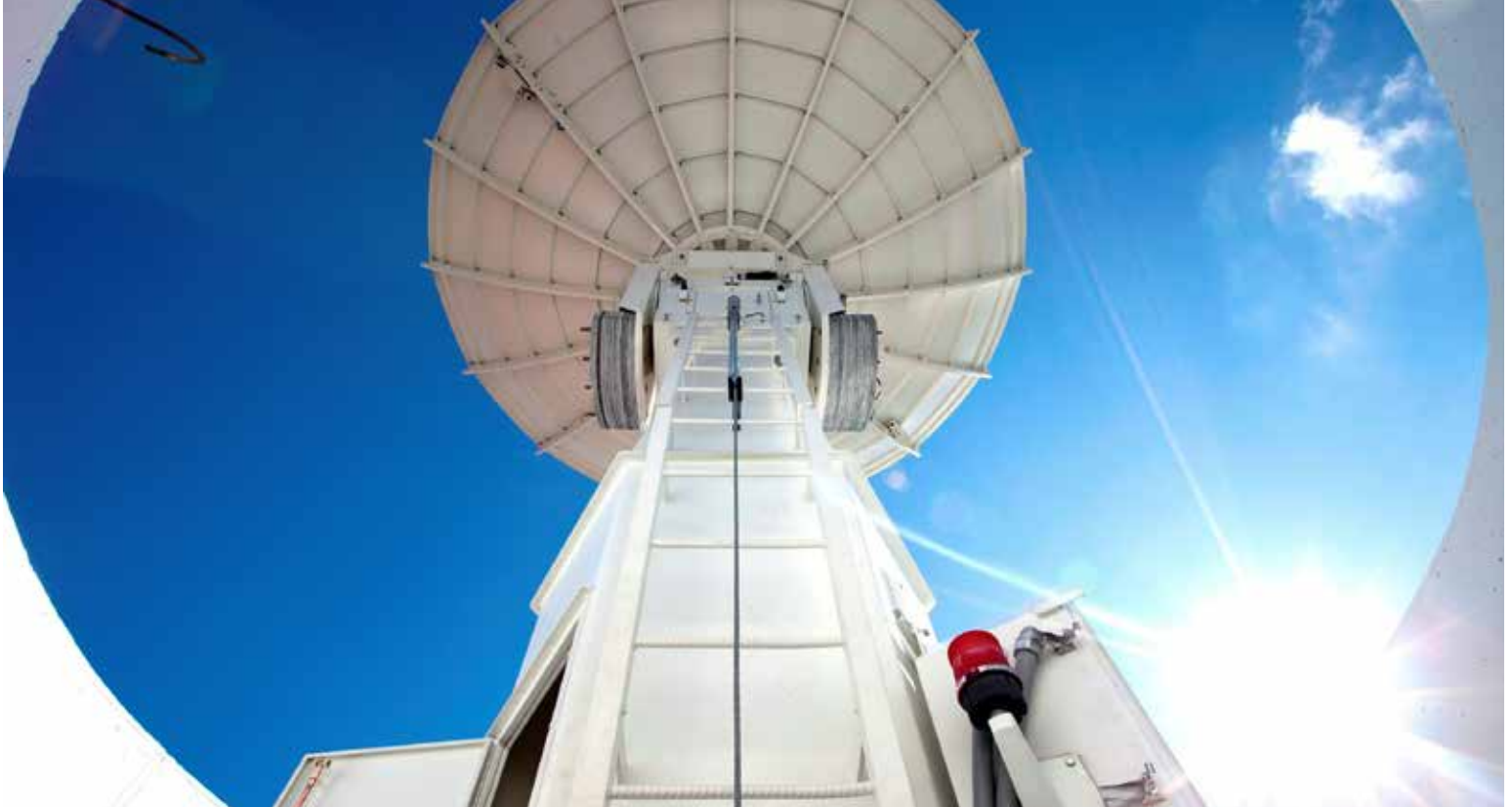
Part of the Kennedy Uplink Station, the S-band ground tracking system at Kennedy provides crucial tracking and communication capabilities following liftoff of SLS and Orion.
