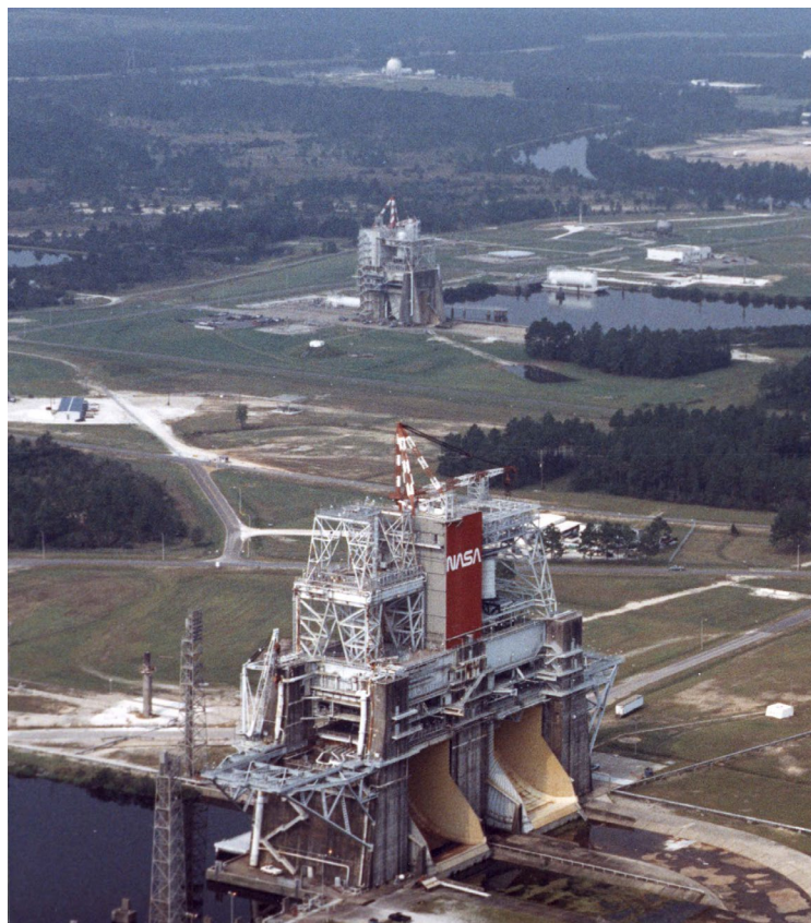
NASA Stennis provides unique facilities for testing SLS RS-25 engines and controllers. The B Complex, foreground, was used for Green Run testing the SLS core stage.
