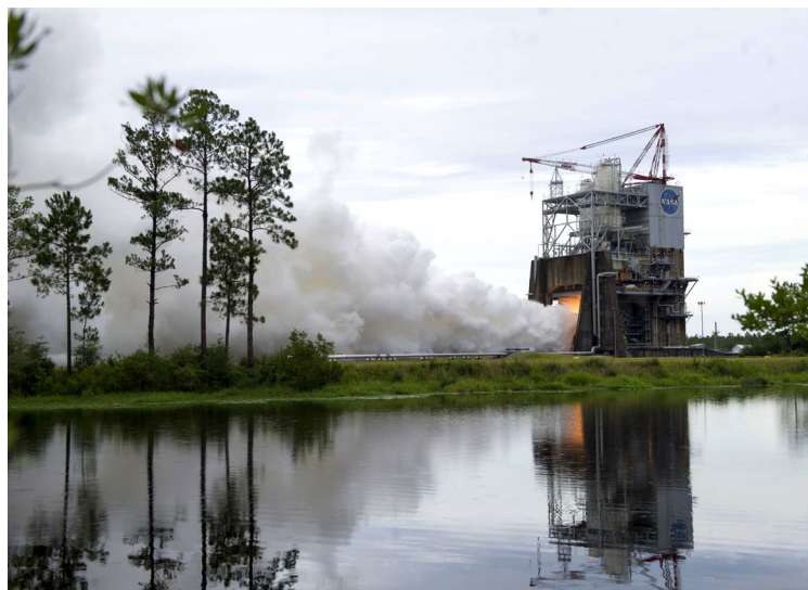
RS-25 engine and controller hot fire testing at Stennis.
