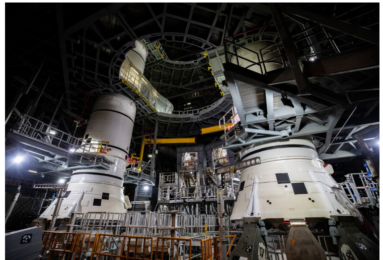
The solid rocket boosters' aft assembly includes the aft skirts with thrust vector control system inside that helps steer SLS during ascent. The entire weight of the SLS vehicle goes through the aft skirt structures.
