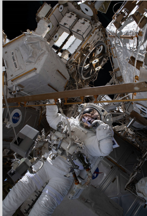
Spacewalk to Upgrade ISS Battery
