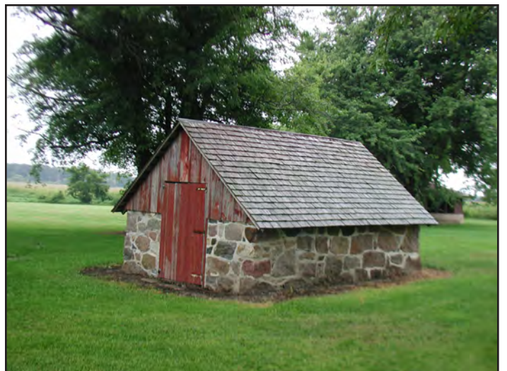
Stone building housing well components at Split Rock Park.
