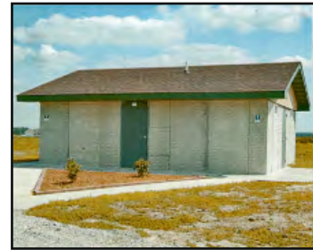
Shower house at McGowen
