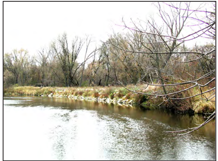
Bank stabilization at Chickasaw Park on the Little Cedar River. This was part of a fish habitat project.
