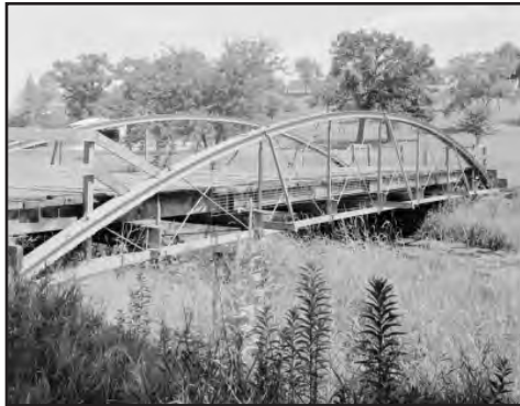
Historic Bridge at Pilot Grove Park
