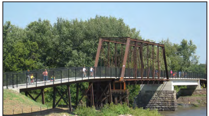
Main bridge on Union Bridge Trail.
