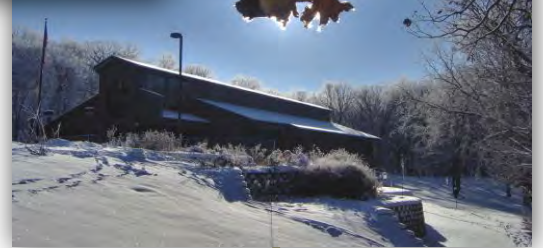
Pecaut Center - Woodbury County
