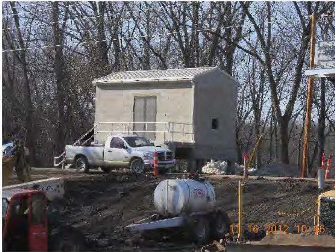
Control Building Complete
