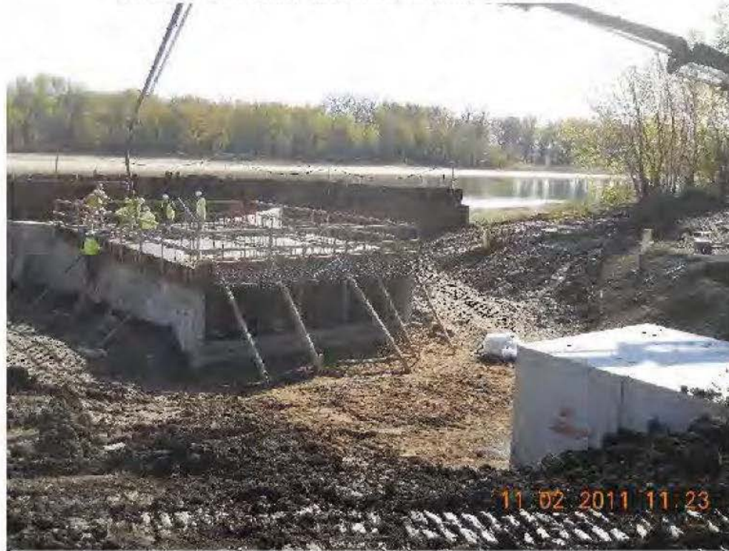
Pump Station raised slab concrete pour. Note Box Culverts Placed.
