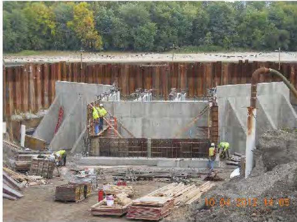
Pump Station receiving chamber wall reinforcing steel tying and form placement
