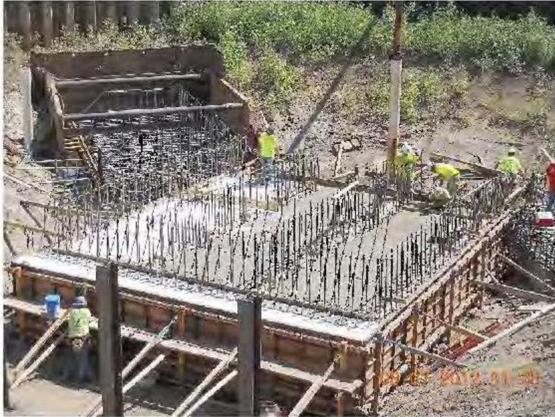
Pump Station foundation concrete finishing
