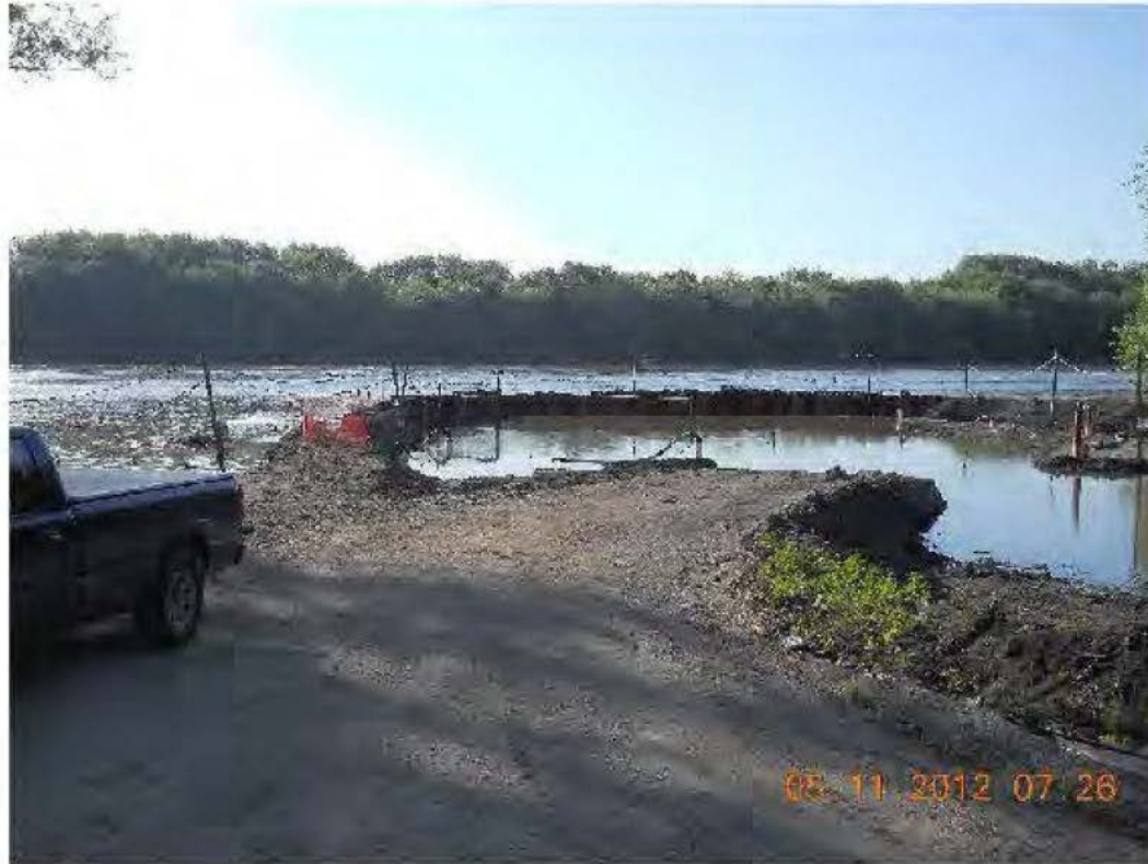
Illinois River flood level in Havana Pool at 14.5 feet in Pump Station Area
