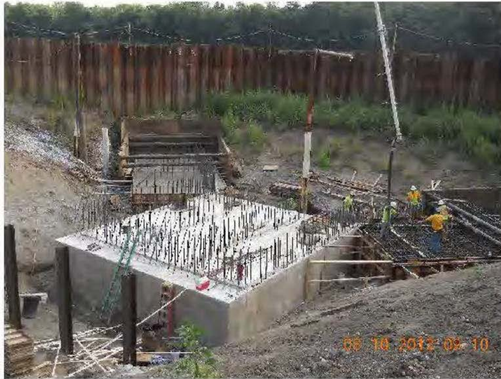
Pump Station Wing Wall foundation concrete pour on August 10
