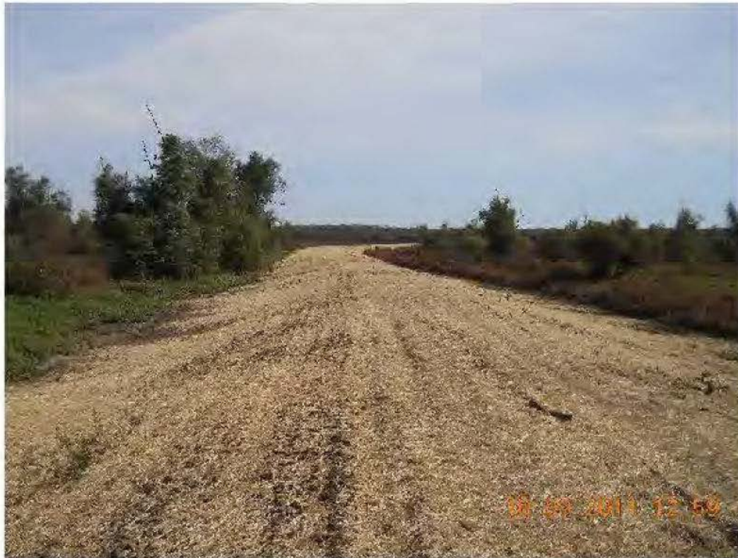
Overflow Spillway (wet and dry) seeded looking toward Goose Lake and River
