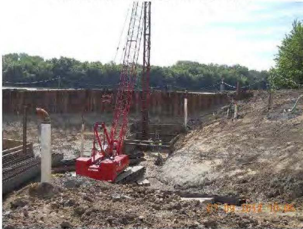
Pump Station H Pile Installation Starts
