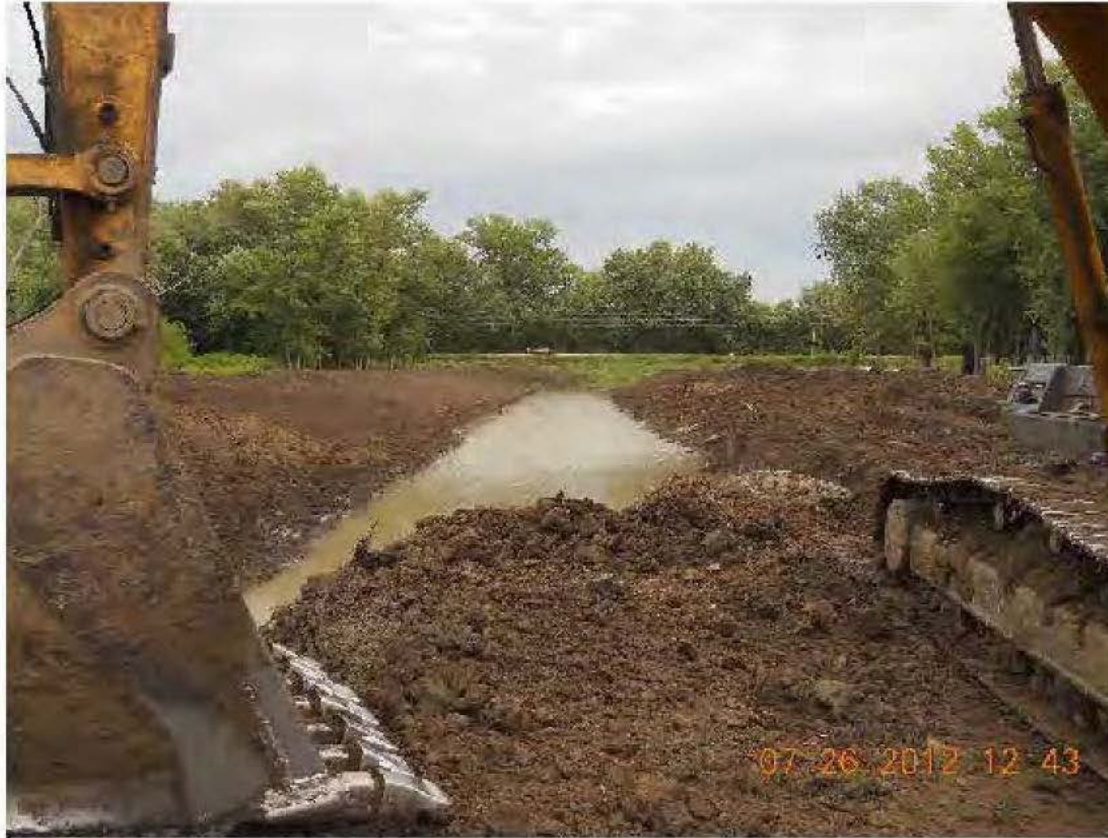
Discharge Channel progress to Station 20+00 looking toward Banner Dyke Road
