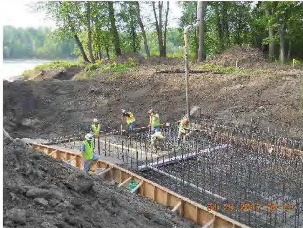
80 cubic yards of concrete poured for Outlet Foundation.
