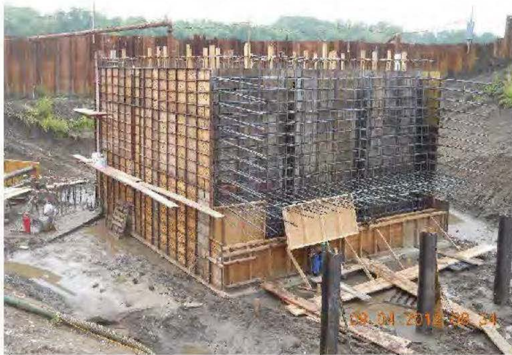
Pump Station chamber wall forms being set. Backfill around foundation complete
