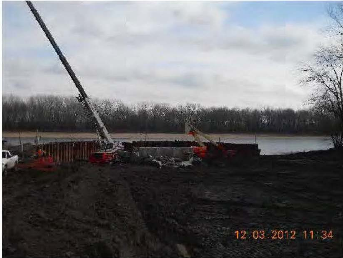
Pump Station Area Clean-up and pulling/abandonment of dewatering wells
