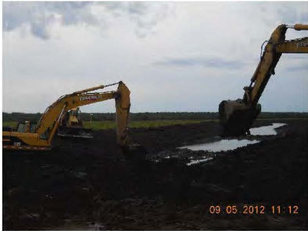
Discharge Channel excavation progress to Station 54+00
