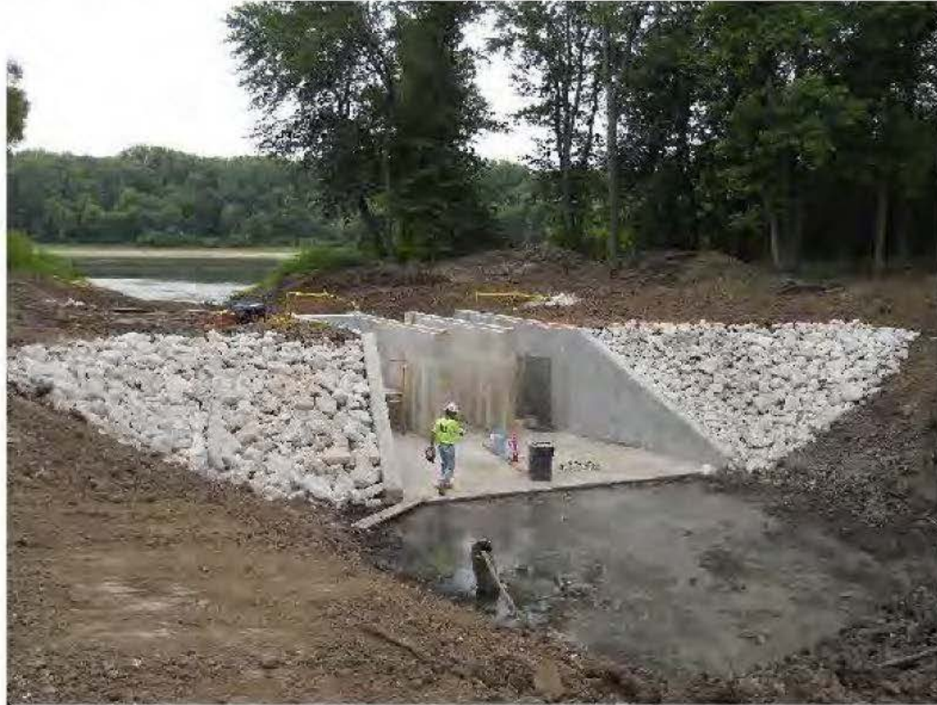
Natural Spillway Outlet Structure after placement of riprap upstream
