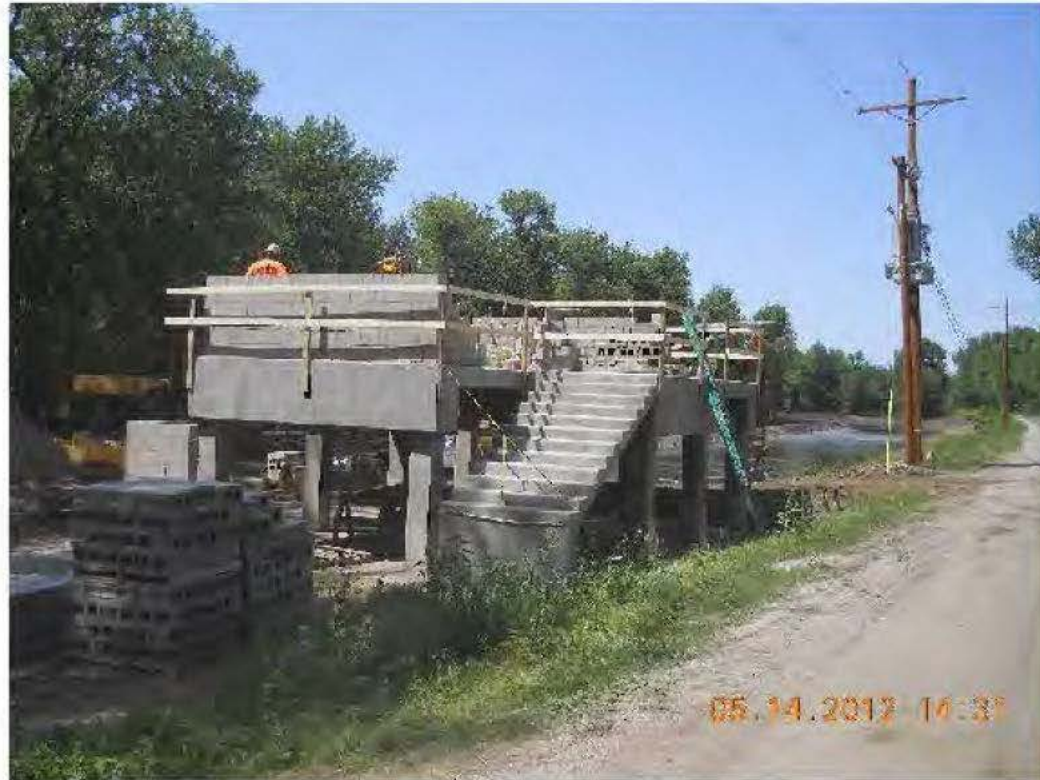
Control Building Masonry Walls being constructed.
