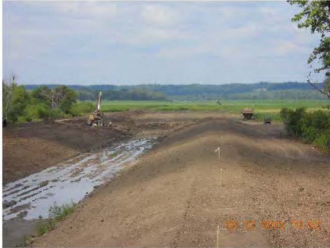
Discharge Channel Excavation and Construction at Station 20+00
