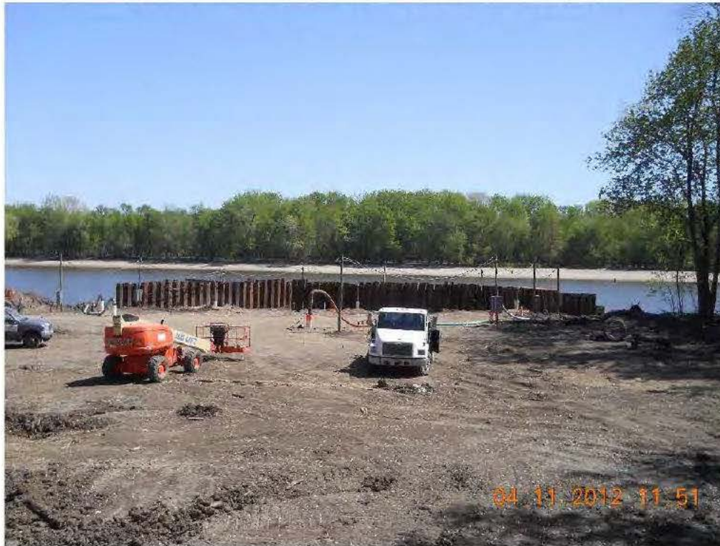
Pumps Station dewatering well installation complete. Waiting on Temporary Power Connection
