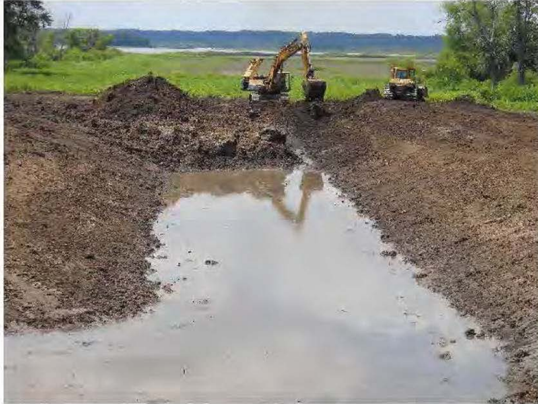
Discharge Channel excavation continues. Berms being built as work progresses
