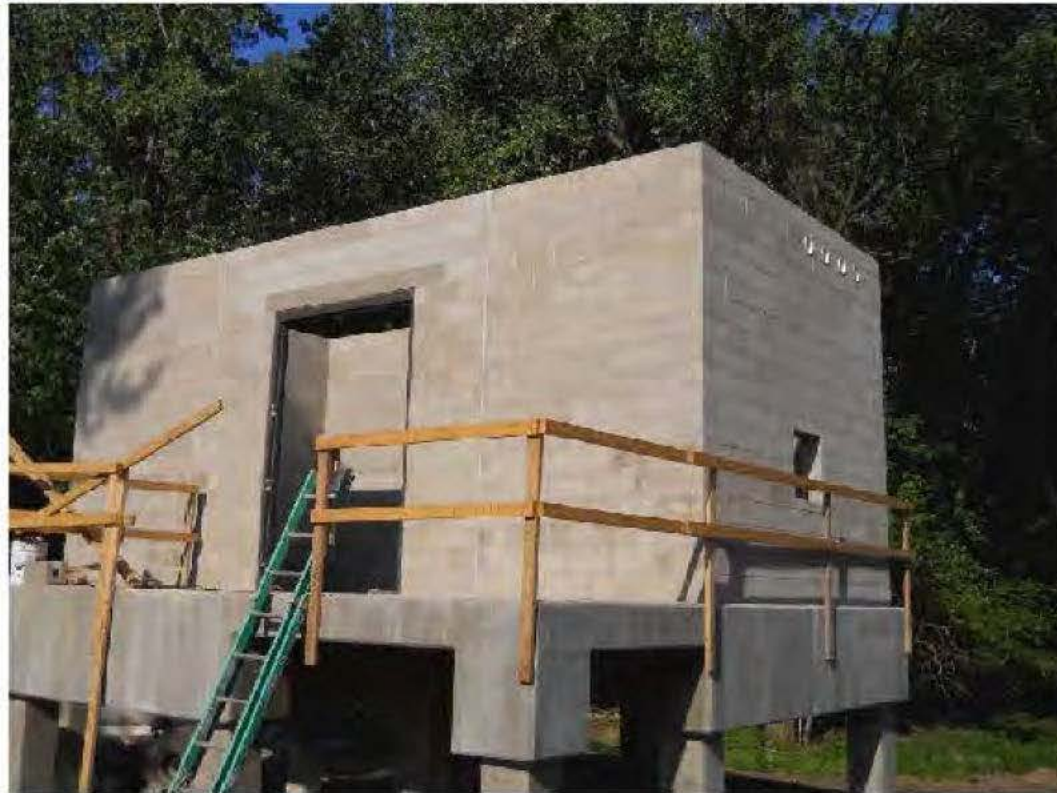
Control Building Masonry Walls complete
