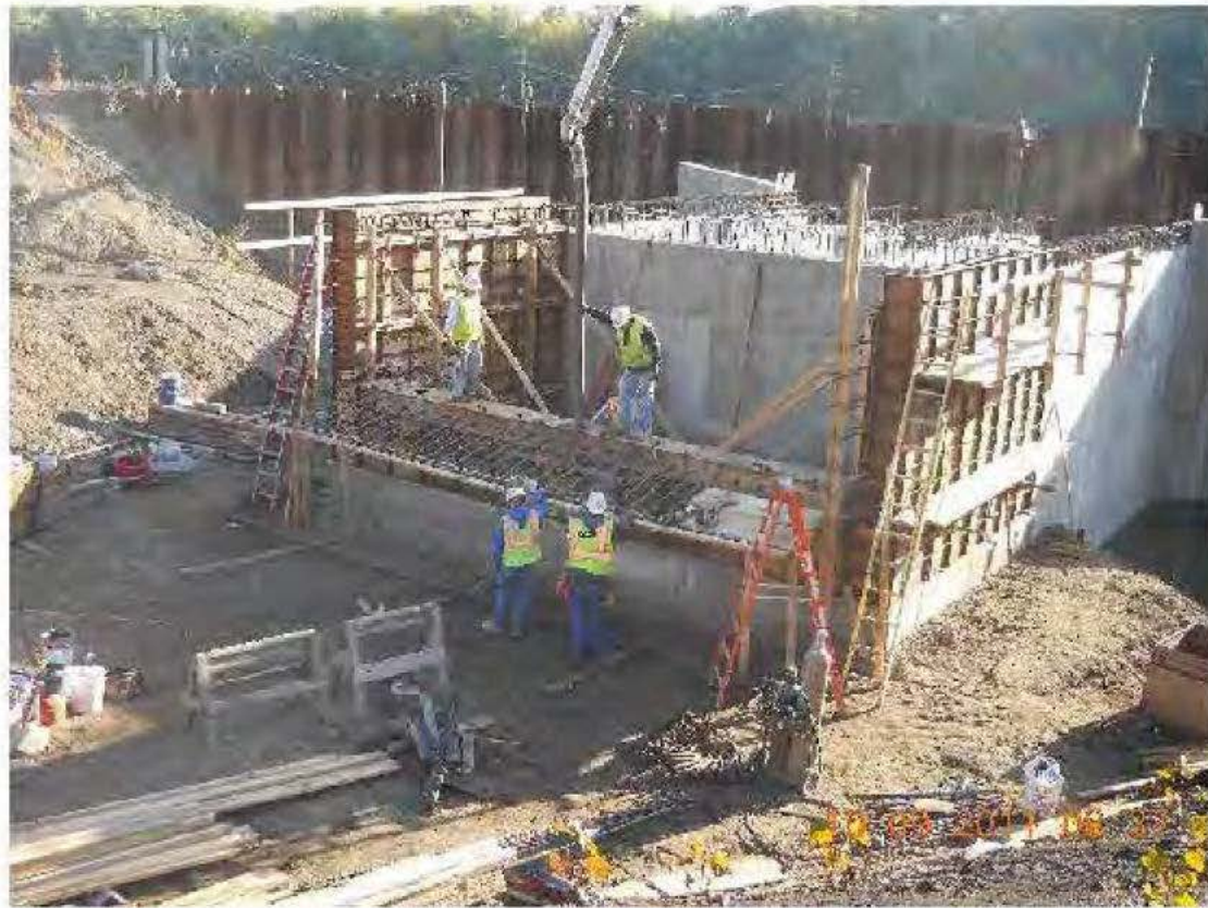
Pump Station Receiving Chamber concrete pour
