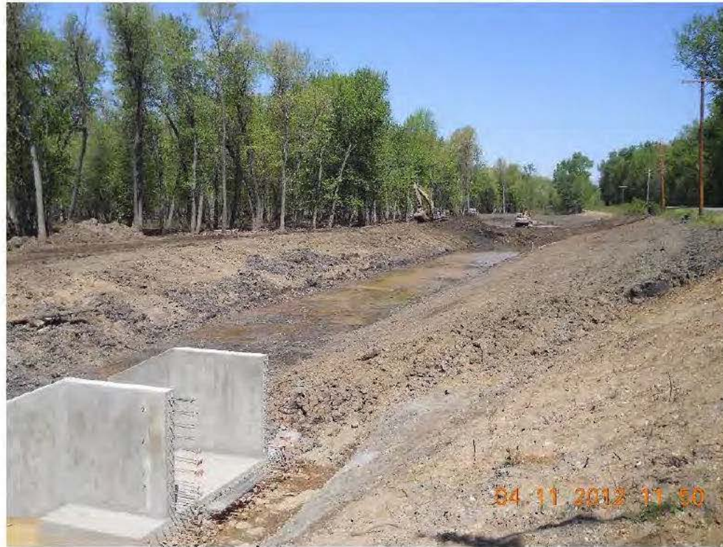
Discharge Channel excavation to Station 4+00
