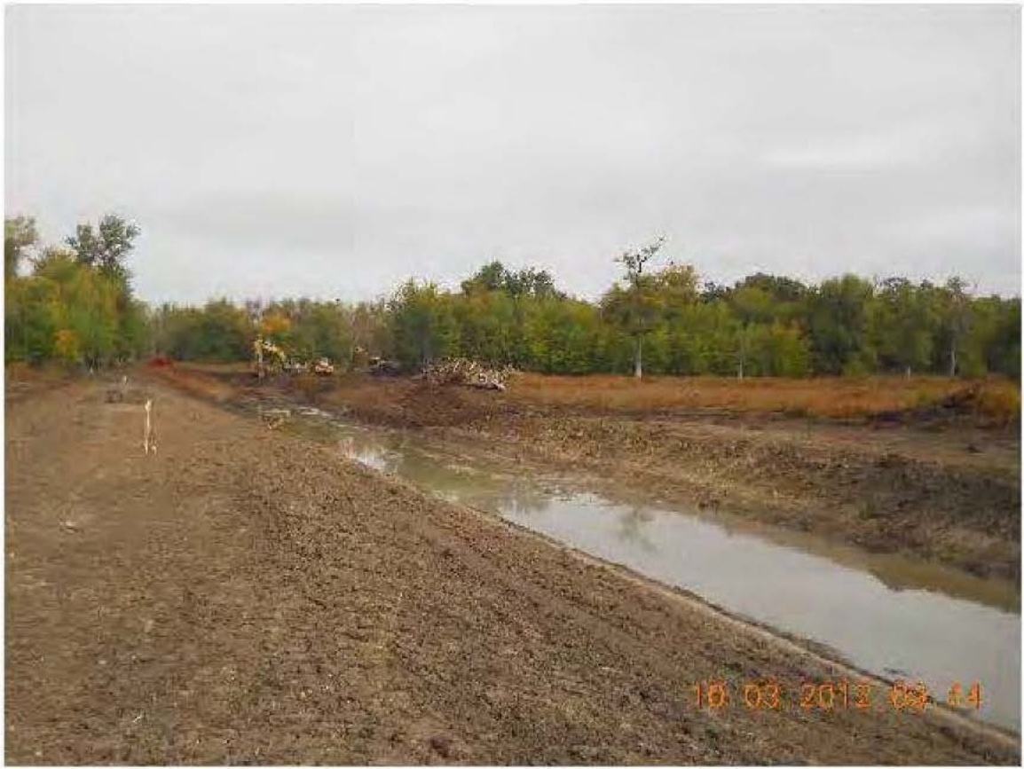
Discharge Channel Clearing and Grubbing complete at Slim Lake
