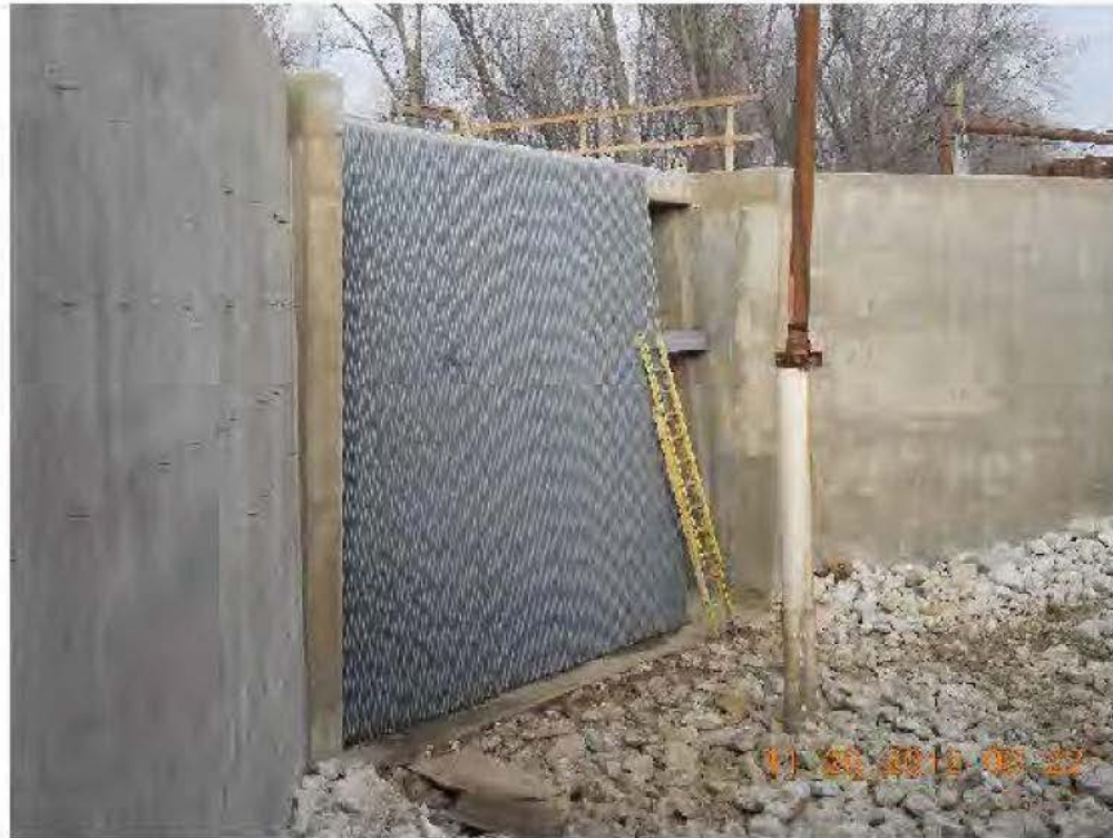
Pump Station Trash Rack Installation
