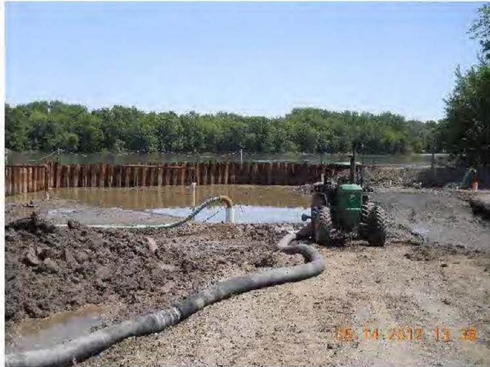
As Illinois River levels decrease, water in Pump Station Area removed
