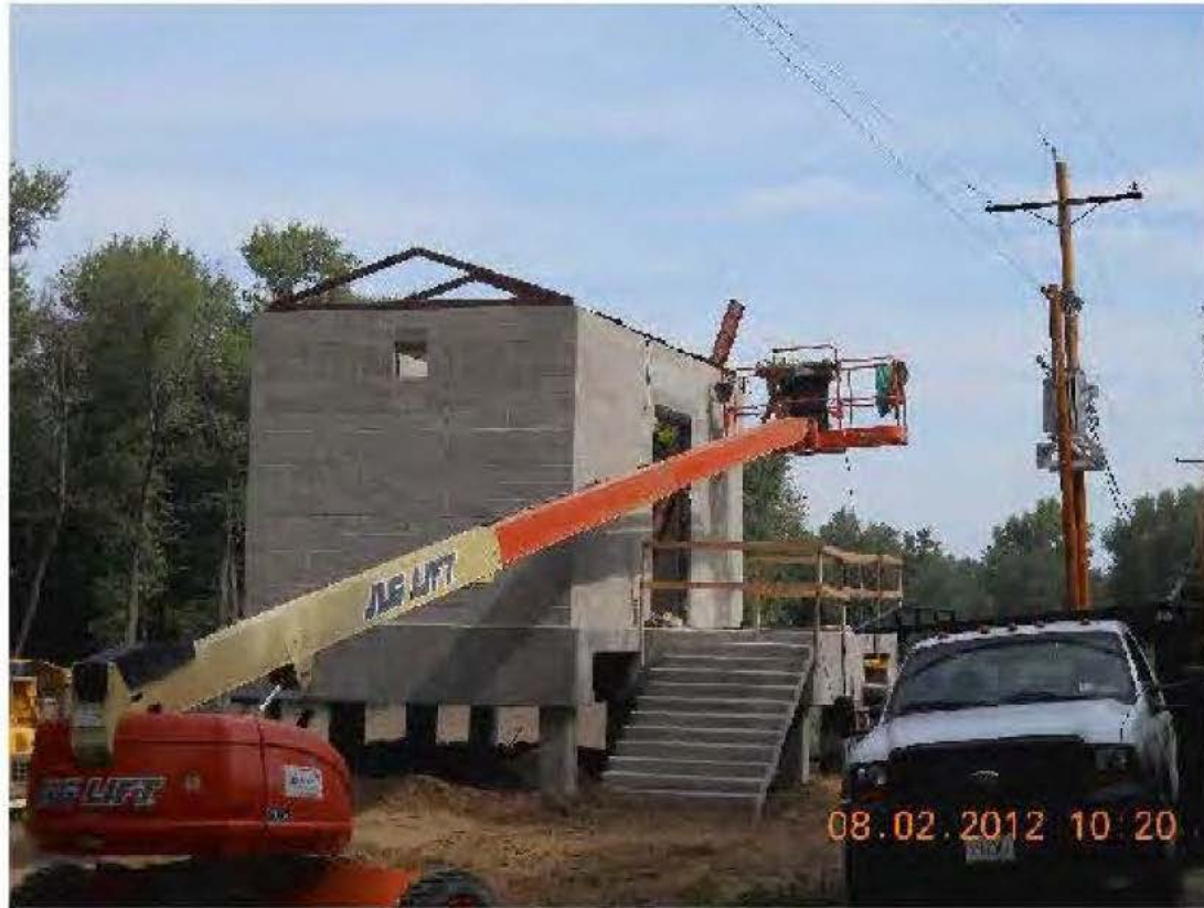
Control Building roof truss and deck installation
