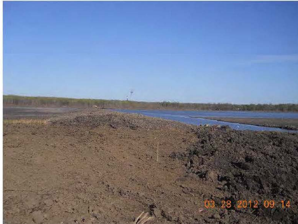
Initial placement of Overflow Spillway from Station 40+00 looking West
