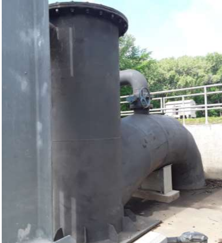
Start of wet test power reading:
