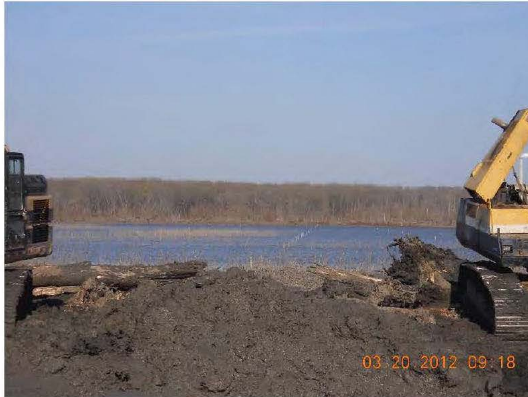
Overflow Spillway alignment stakes across Goose Lake behind equipment
