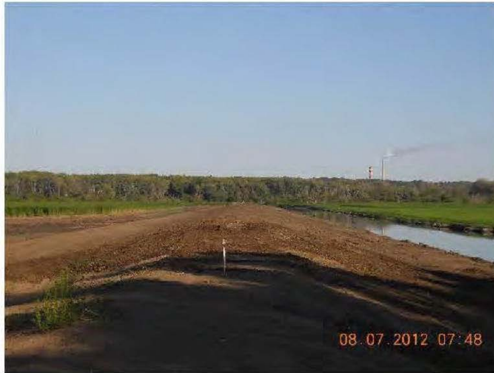
Overflow Spillway in Wet final grade. 2012 construction complete
