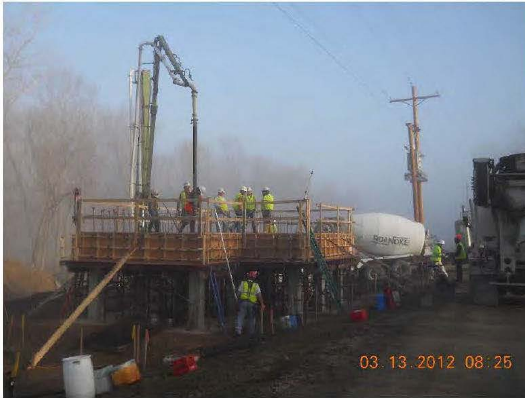
Control Building deck and support beam concrete pour in progress
