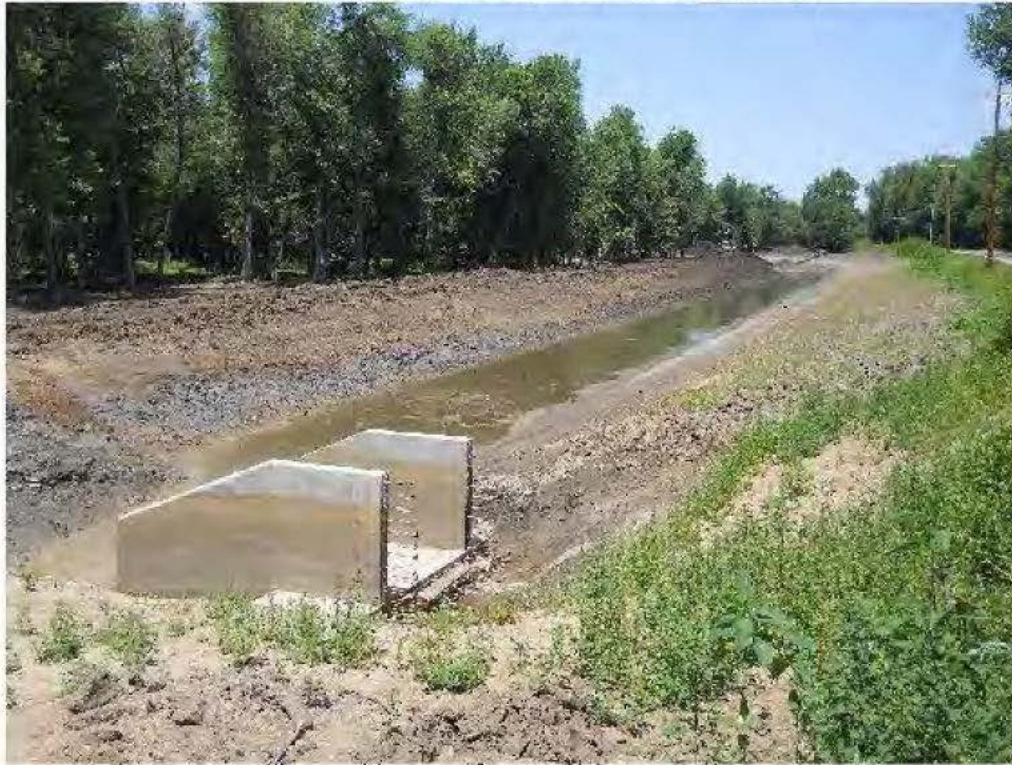
Discharge Channel drained after May Flooding
