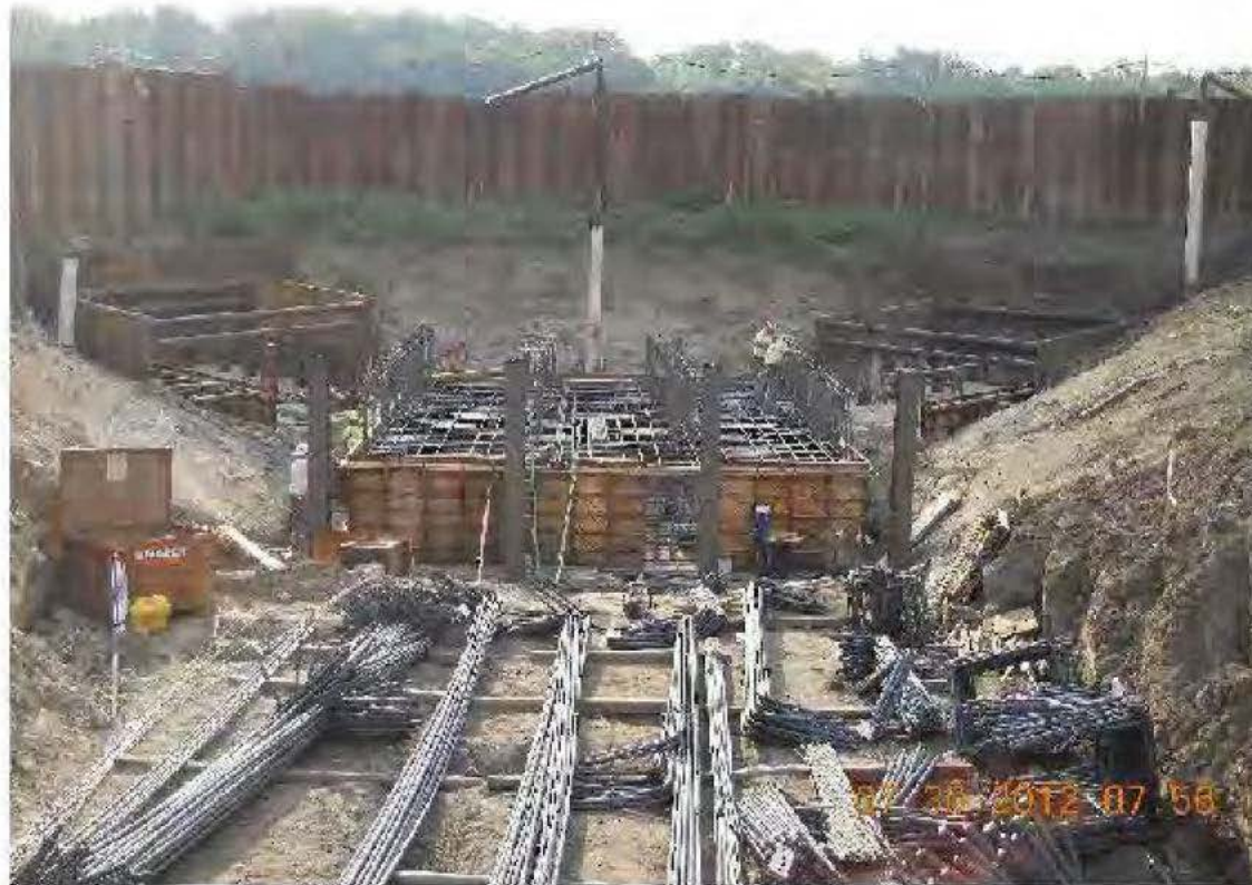
Pump Station foundation reinforcing steel installation
