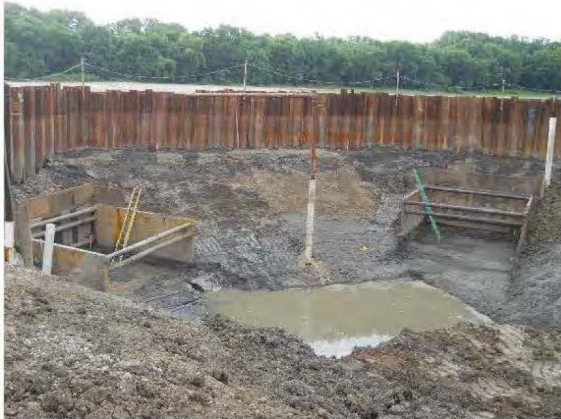
Pump Station Area during foundation excavation
