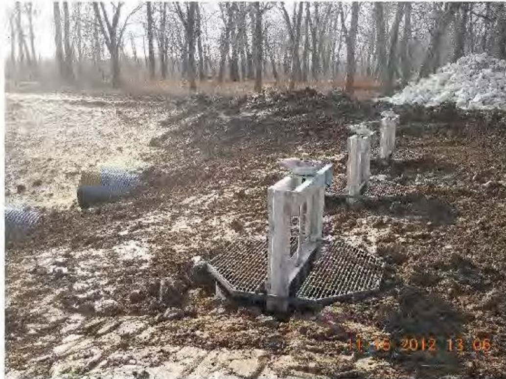
48-inch Gates and CMP discharge to Rice Lake complete in area of Eagle Nest.
