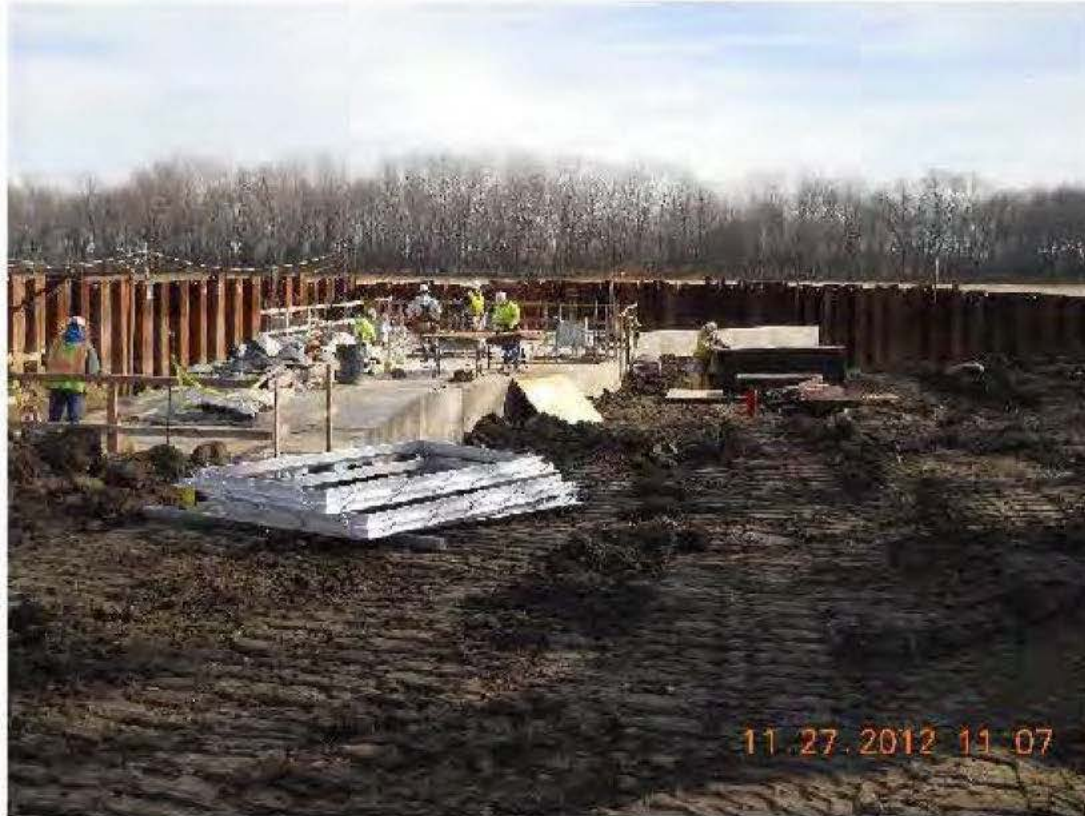
Pump Station Raised Slab Modification Work
