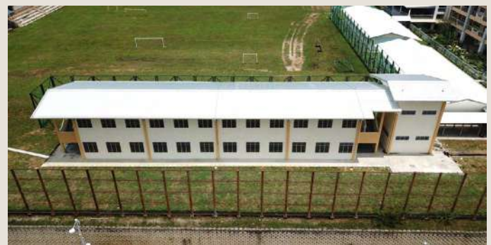
Completed classrooms built using our MBS technology
