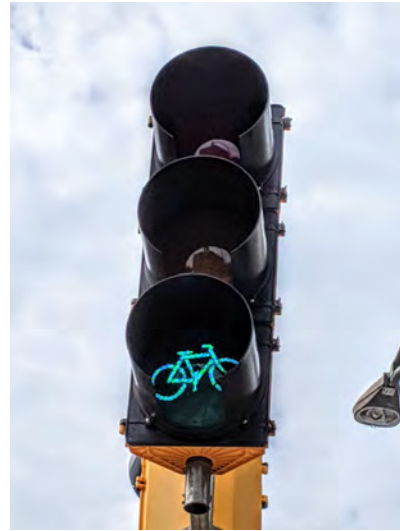
Figure 53 - Bicycle signal at Second Ave / Wayne Ave & Colesville Road (MD 384)
