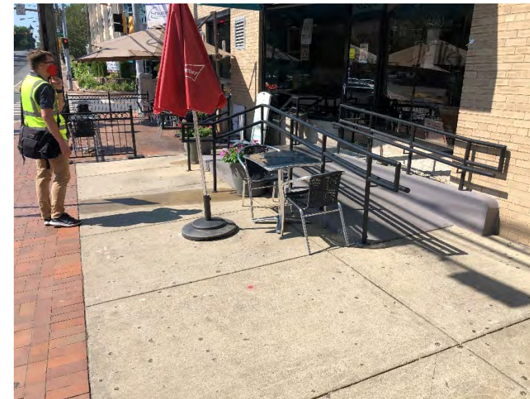
Figure 64 - Existing ADA ramp access to restaurant/cafe on the NW corner of Fenton Street and Silver Spring Ave
