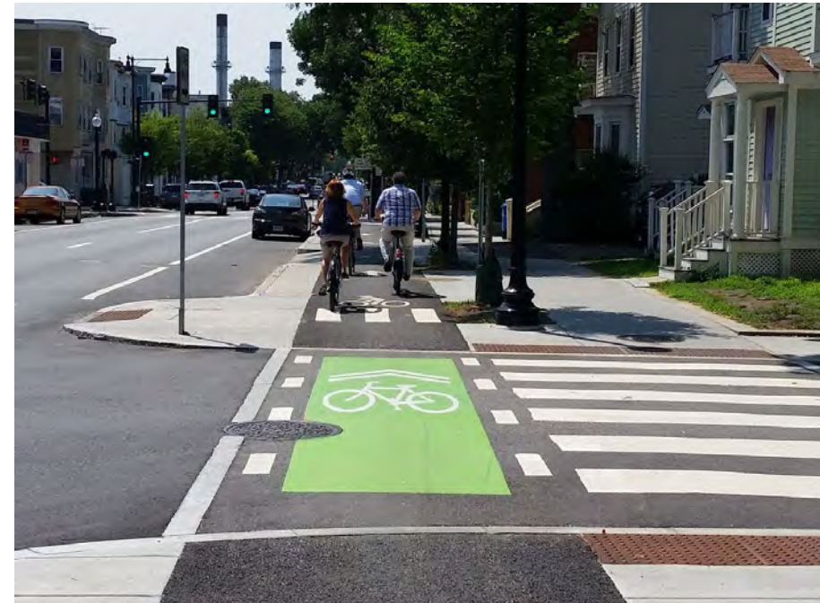
Figure 60 - Example treatment at side street intersection with a one-way cycle track in Cambridge, MA.
