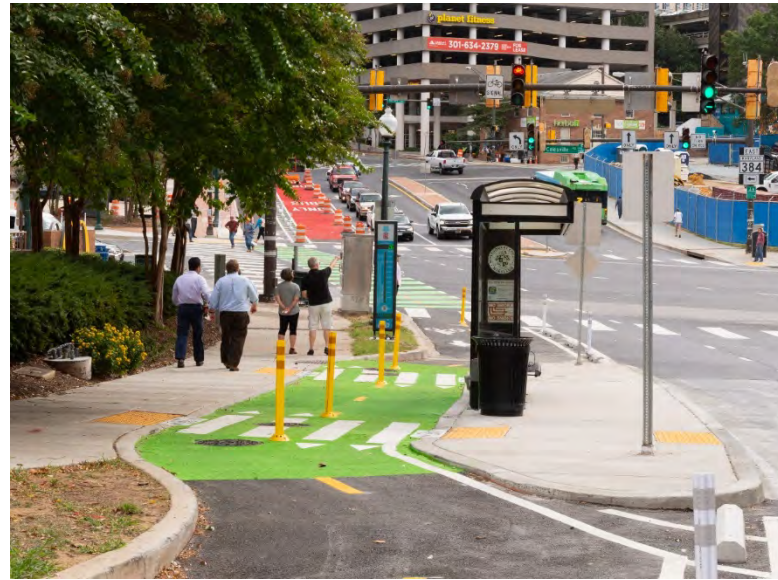
Figure 66 - Floating bus stop located at Second Avenue, north of Colesville Road, Silver Spring, MD.
