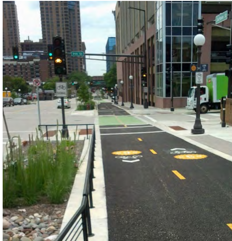
Figure 56 – Two-way cycle track with MUTCD experimental flashing yellow signal treatment in St. Paul, MN.
