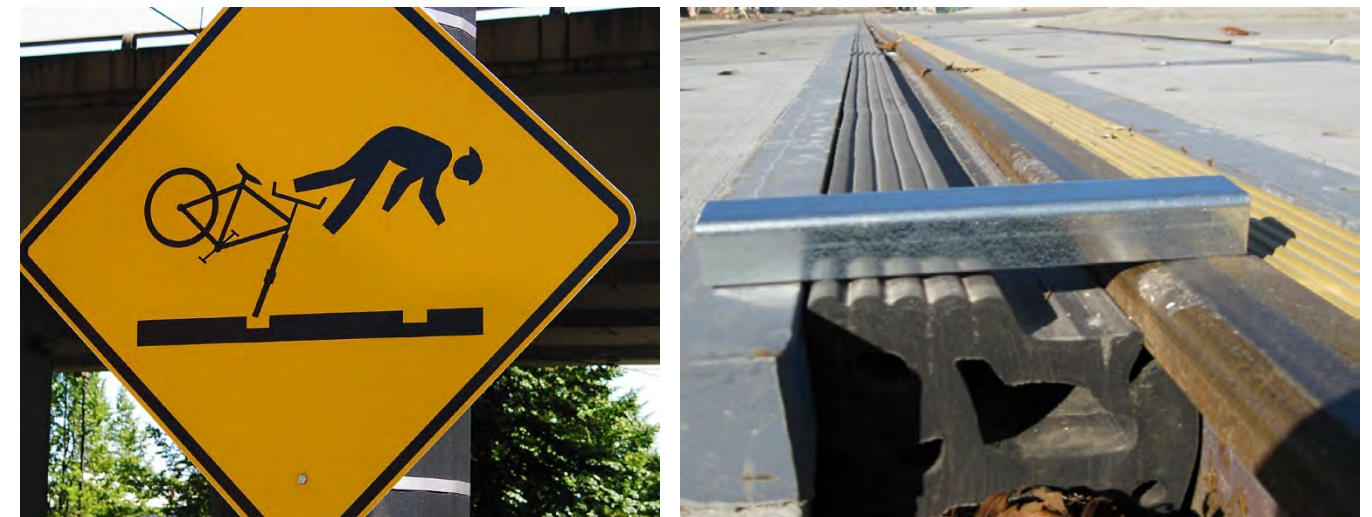
Figure 65 - Example caution signing from Portland, OR used to warn bicyclists of the hazard associated with riding parallel to light rail tracks in the roadway (left); Example of flangeway filler used to fill gap between track and pavement (right).
