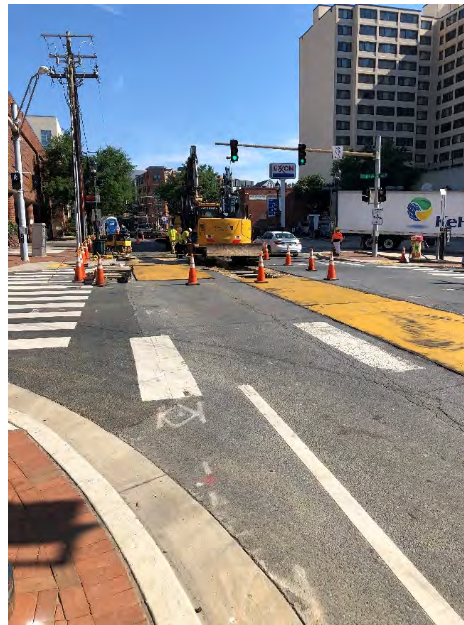
Figure 11 - PEPCO undergrounding work at Fenton Street and Thayer Avenue in July 2020.
