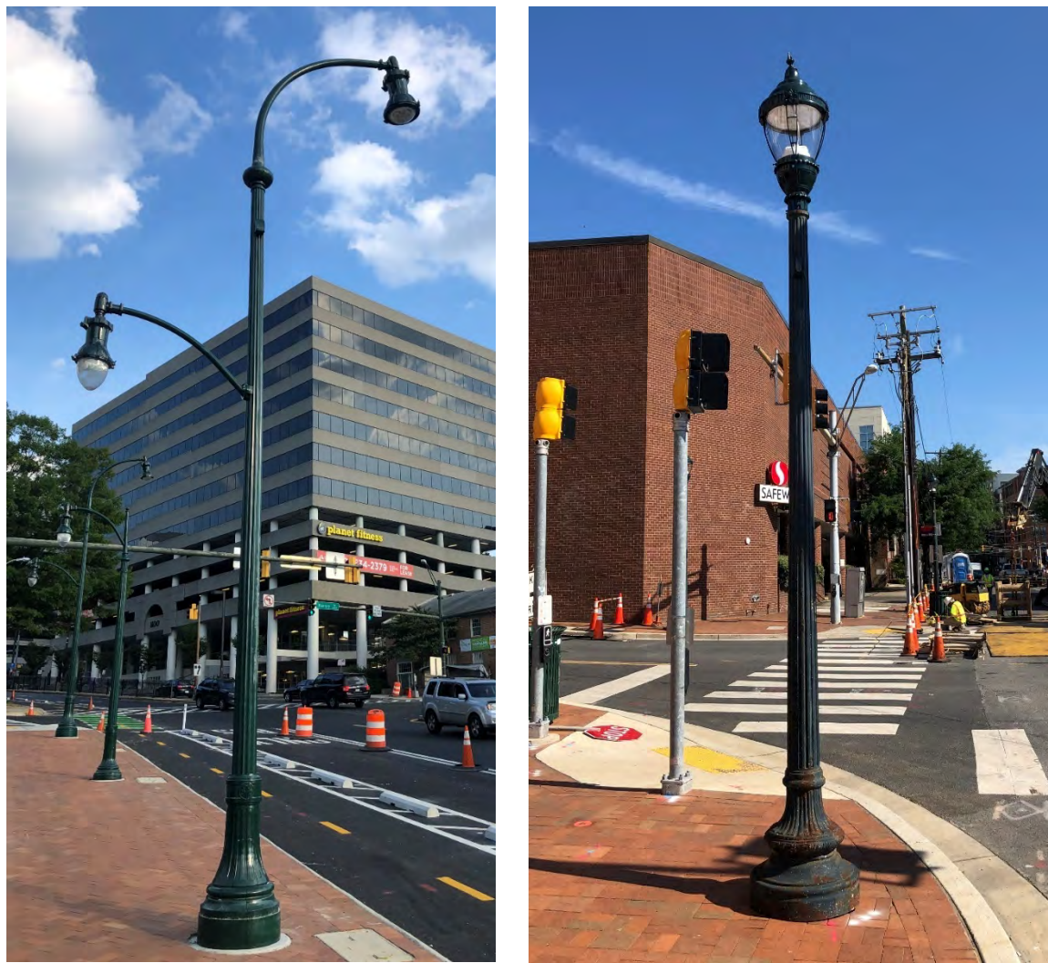
Figure 61 - Silver Spring CBD standard lighting: Dual Combination teardrops and Pedestrian teardrops (left) and Washington Globe pedestrian light poles (right).
