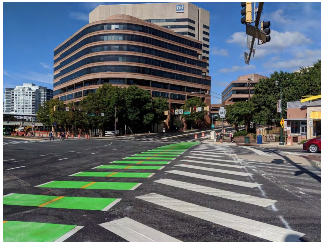
Figure 57 - Green paint conflict zone at Second Ave / Wayne Ave and Colesville Road (MD 384)
